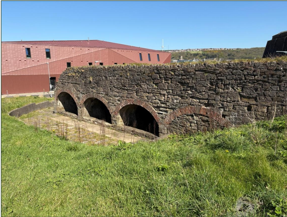
Photo 20: View south of the tramway bridge associated with the Wellington Pits transporting coal directly to the harbour (HER 4173), seen on the 1 st Ed OS Map 1861.
