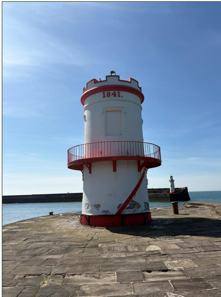
Photo 14: N Pier lighthouse 1841. View west towards West Pier Lighthouse (Grade II listed, NHLE: 1086806 ).
