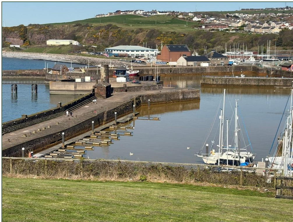
Photo 22: Close up shows orange ochre contamination around all walls within the Inner Harbour.
