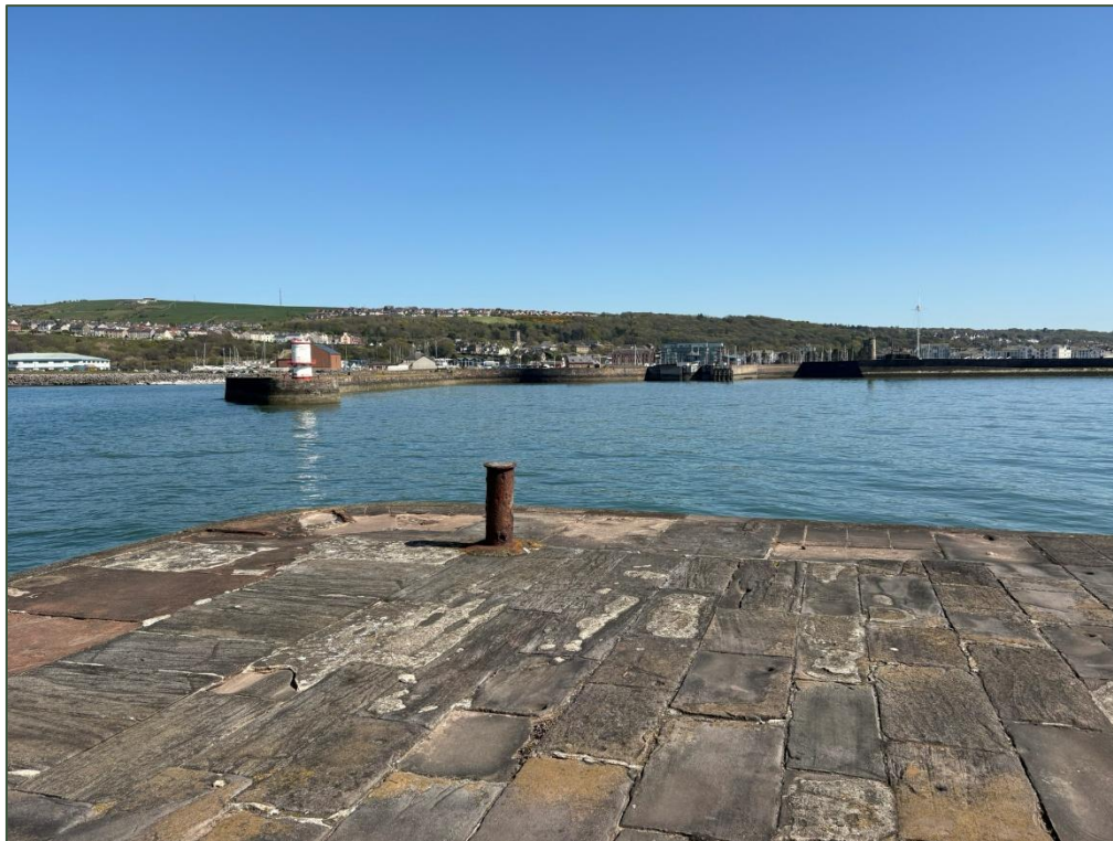
Photo 17: View southeast from west pier lighthouse towards the site. No indirect impact of the ochre contamination or the proposed pipe installation was identified during the site visit.
