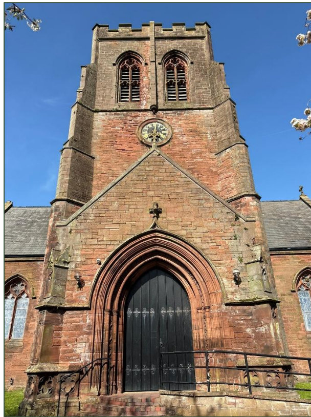
Photo 28: Tower Chapel of St Nicholas (Grade II listed, NHLE: 1038534 ).
