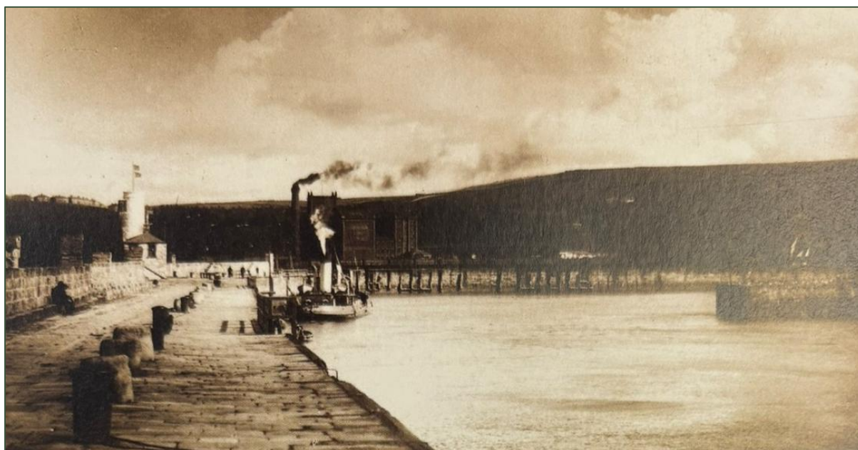
Plate 17: Old Quay, view north. The eastern elevation, although shows some sloping, appears more exaggerated today as seen in Photo 16 .
