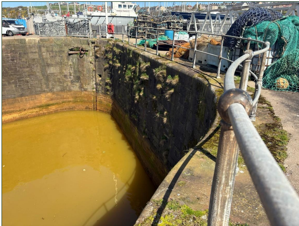
Photo 5: View from Queens Dock lock along the Old North Wall (Grade II Listed, NHLE: 1038936 ) on the Inner Harbour side. Note historic cast iron features within the corner of the harbour wall. Metallic features could be affected by the iron ochre contamination.
