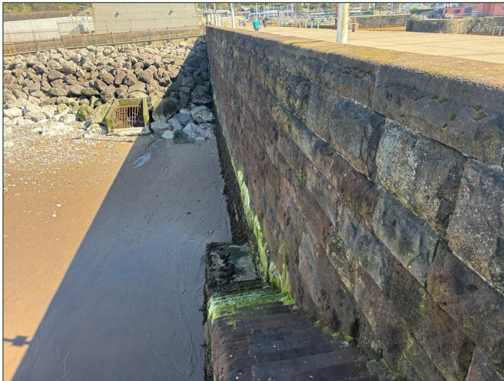
Photo 9: Proposed pipe route through Old North Wall (NHLE: 1038936 ) and the existing UU sewer pipe. Option 2 within Section 2 of this report suggests that the proposed pipe could attach to the UU sewer pipe and discharge directly onto the beach from there, depending on Ground Investigation results.
