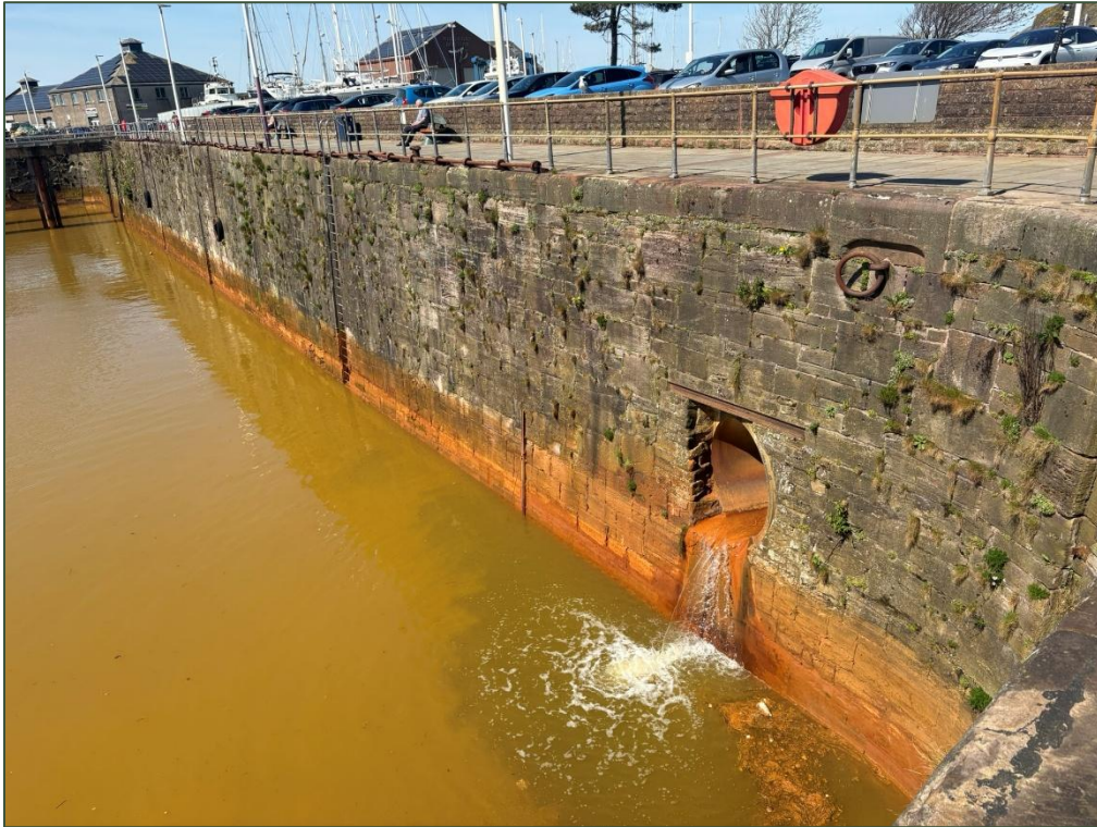
Photo 1: Mine water outfall discharging iron ochre-contaminated water into Whitehaven Harbour. The resulting widespread ochre staining affects the water, harbour structures and the visual appreciation of Queen's Dock and the Inner Harbour.
