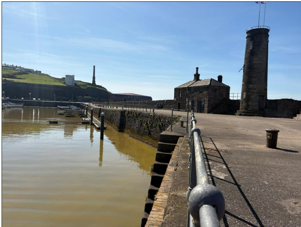
Photo 15: View west from the north-east end of the Old Quay (NHLE: 1004593 ) towards the Grade II listed Watch House (NHLE: 1390499 ), Old Quay Lighthouse (NHLE: 1086805 ) and the Candlestick (HER 43085 ). Iron ochre staining detracts from the appearance of the harbour, reducing appreciation of the historic relationship between the harbour water and the surrounding heritage assets.
