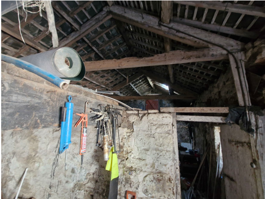
PHOTO 11 BARN 6 SINGLE STOREY ROOF STRUCTURE
