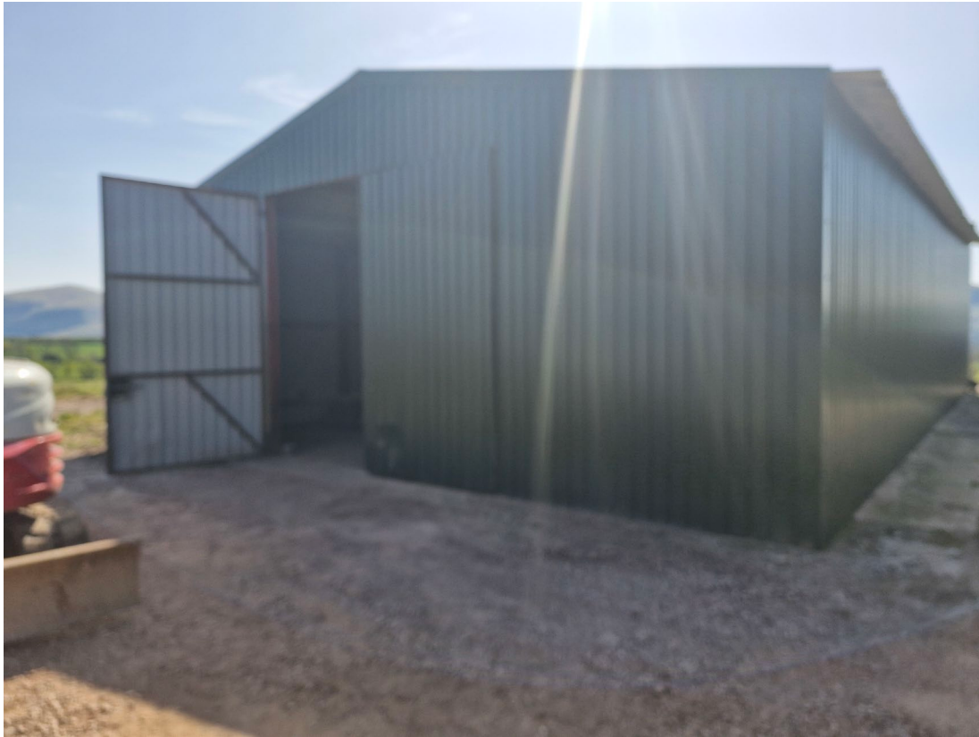
PHOTO 03 BARN 5 FRONT ELEVATION
