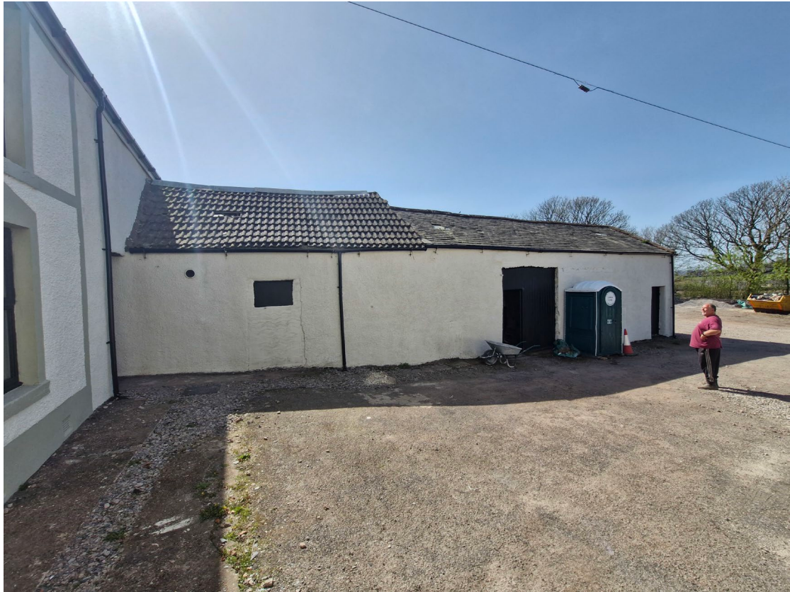
PHOTO 07 BARN 6 FRONT SINGLE STOREY EXTENT
