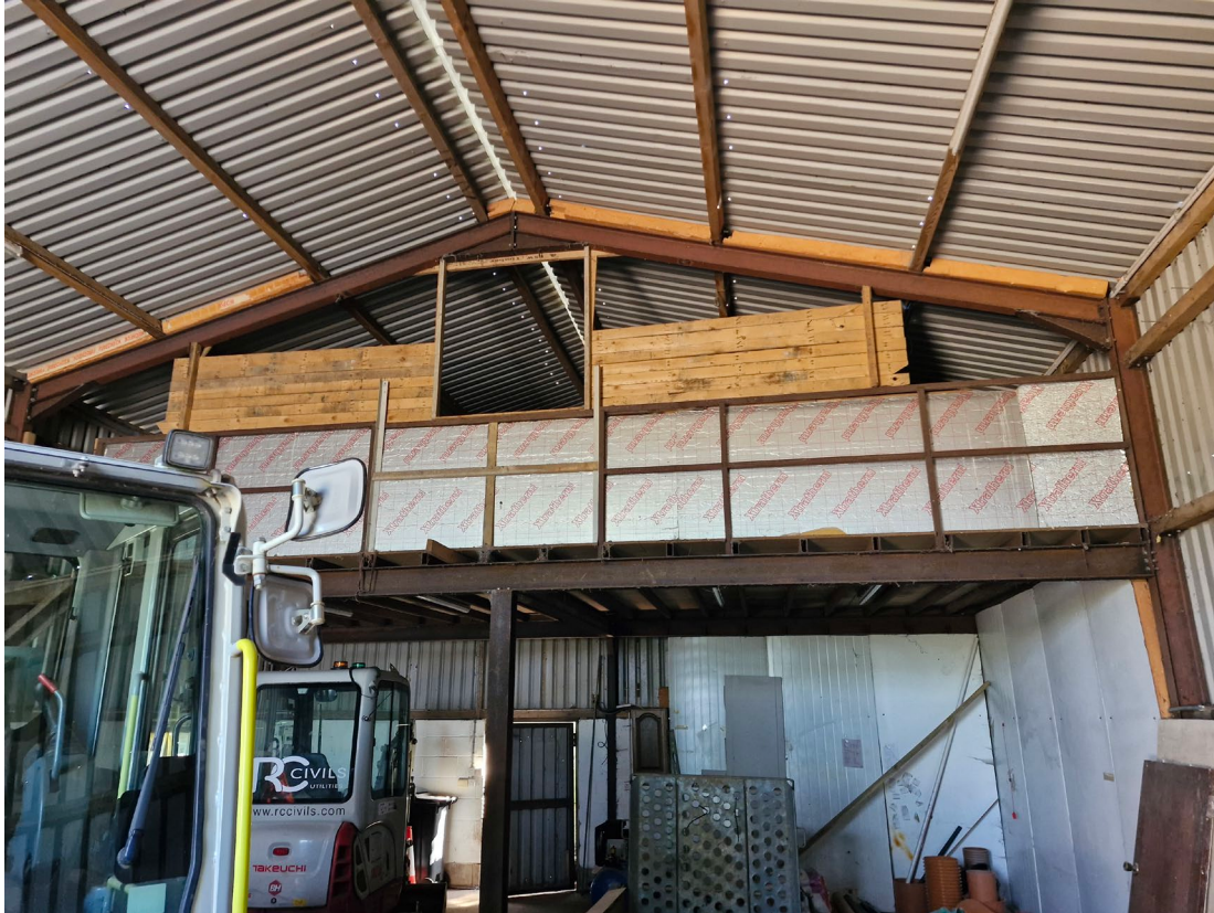
PHOTO 02 INTERNAL VIEW BARN 1
