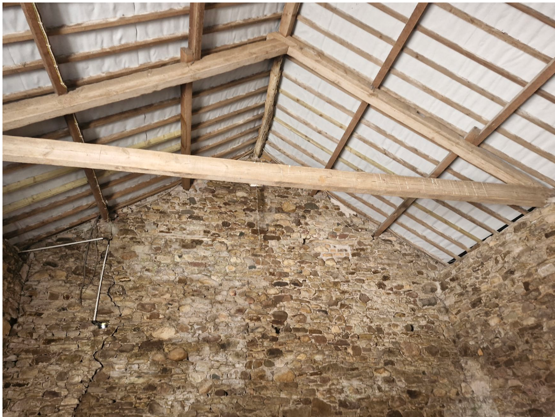
PHOTO 10 BARN 6 INTENRAL VIEW TWO STOREY EXTENT
