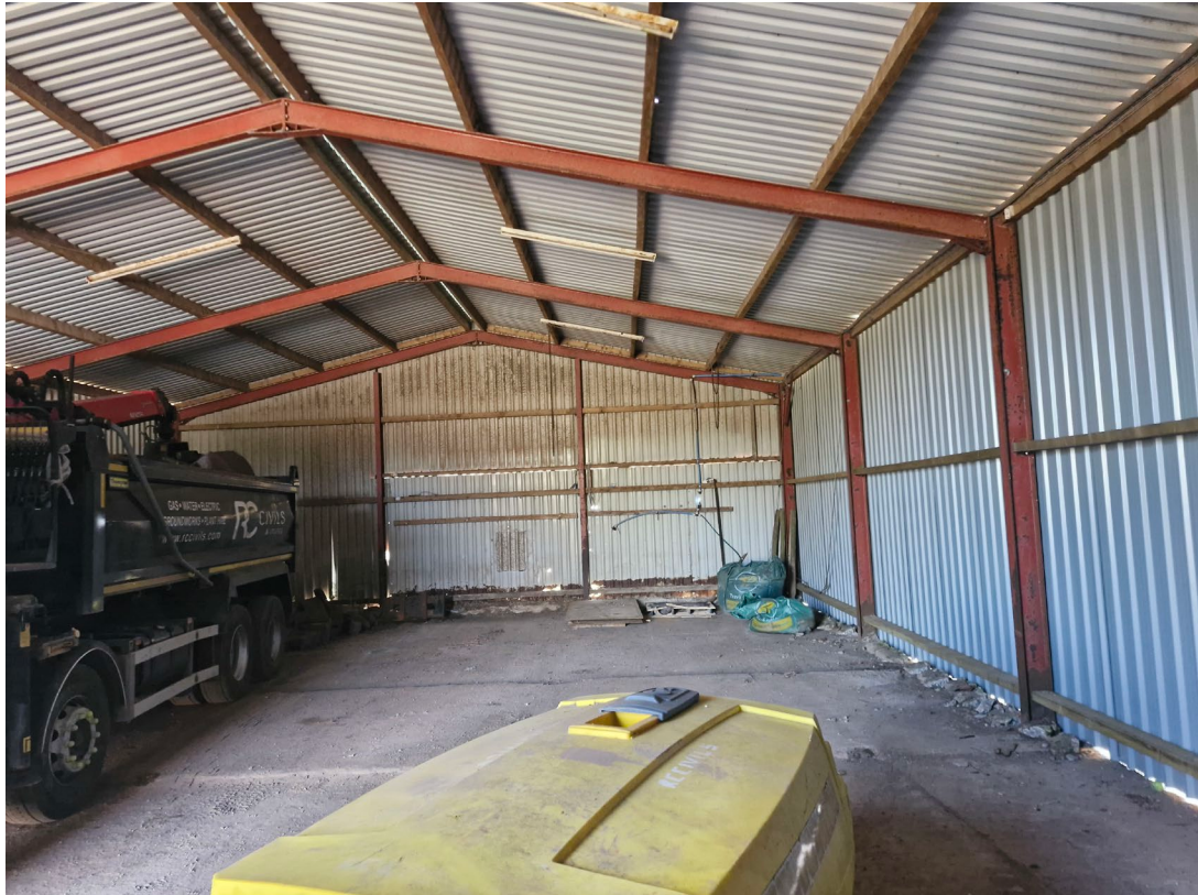
PHOTO 04 BARN 5 INTERNAL VIEW
