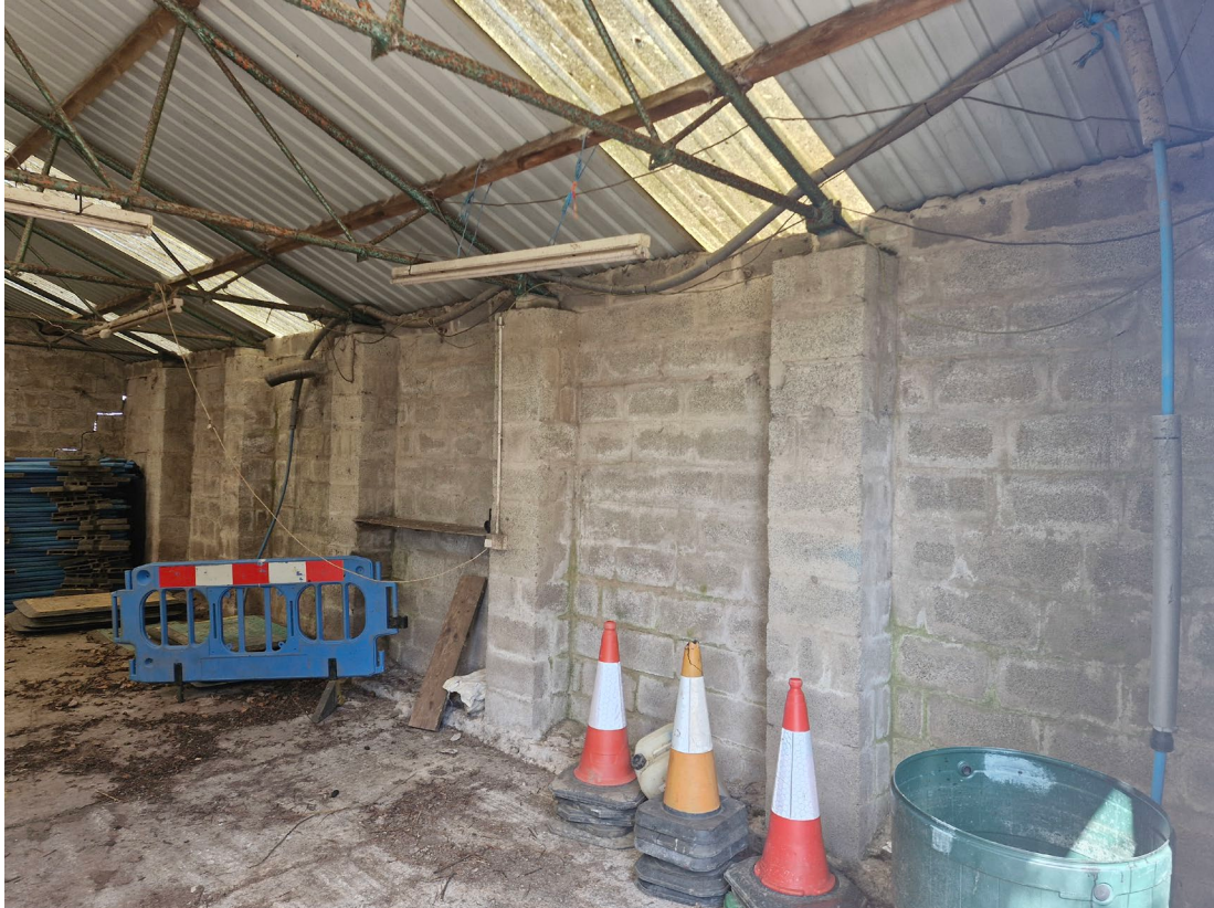
PHOTO 06 BARN 4 INTERNAL VIEW
