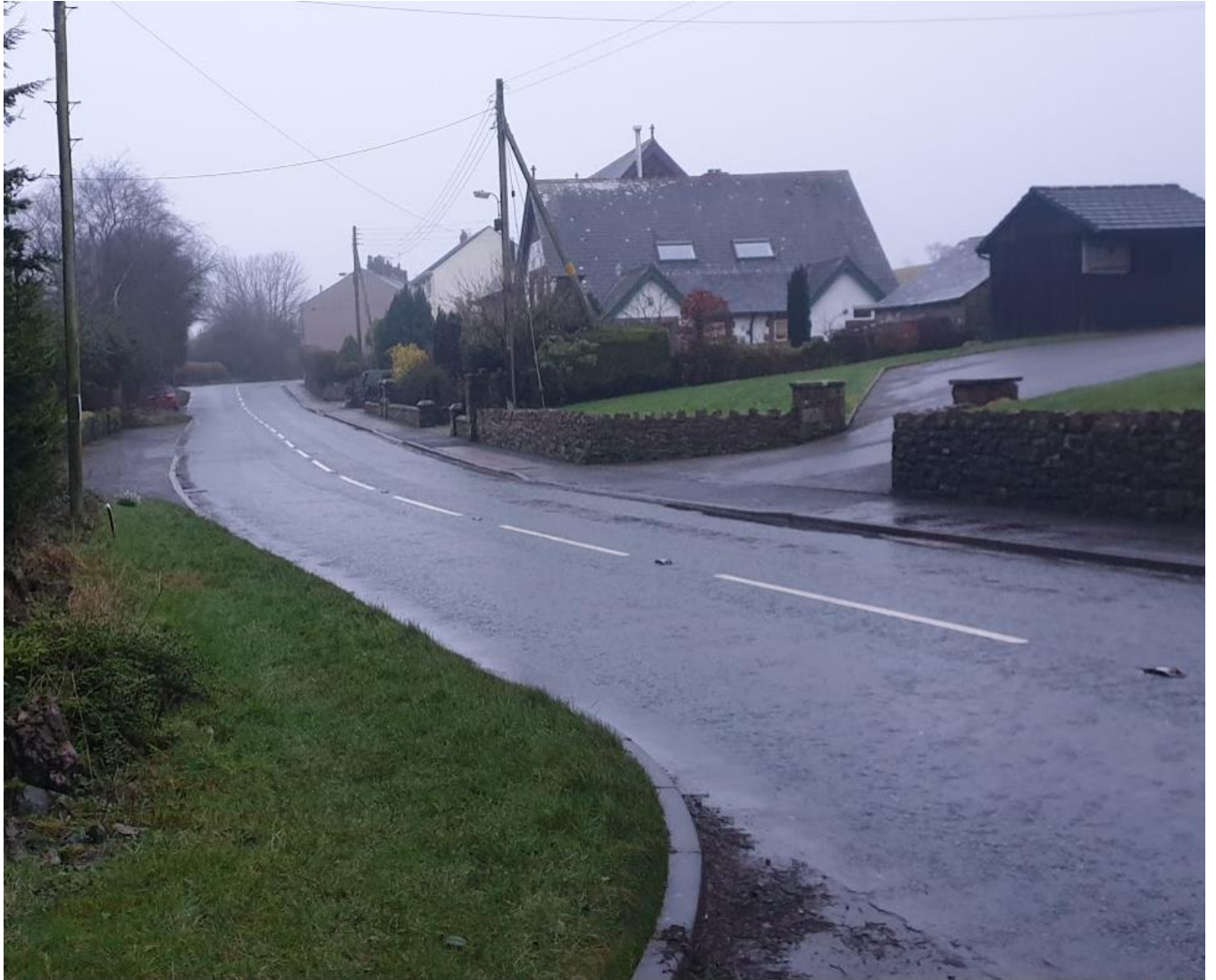
Photo 3 Looking W to Point A
