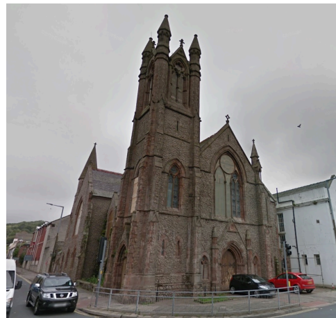
Image of the former Methodist Church building.
