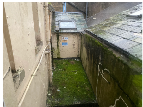
Image of the remaining open area to the rear of Union Hall at 1 st floor level. Note the moss-covered corrugated roof encloses the 'yard' area at ground floor level.
