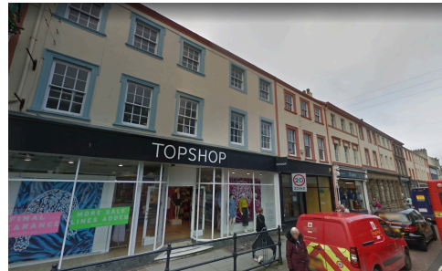
Lowther Street group of attached Listed buildings.
