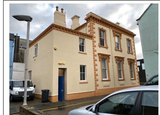
Image of Union Hall with two storey addition fronting Fox Lane, following external decoration.
