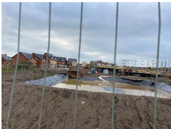
Photo 13 – Construction site pond
