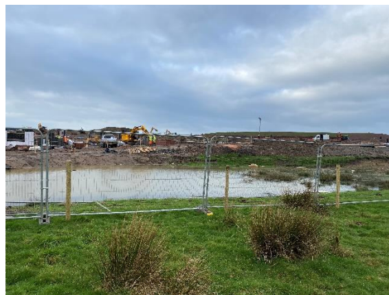
Photo 14 – Construction site pond
