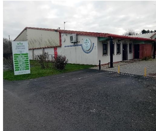
Photo 4: Main building to east of entrance
