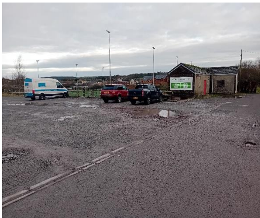
Photo 3: Site overview from entrance
