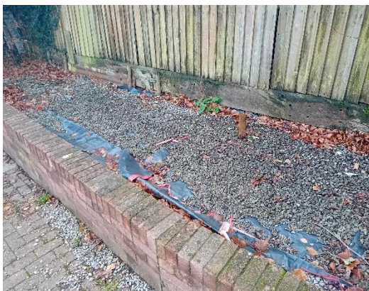
Photo 5: Southern boundary with Misslethwaite Cottage
