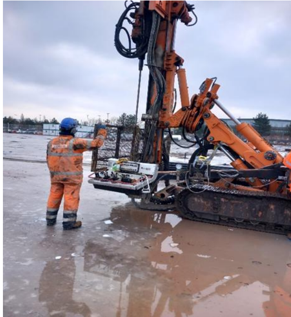
Figure 8: Checking mast is at the correct orientation.
