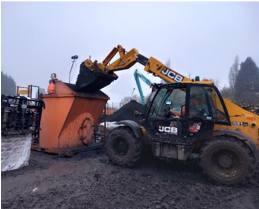
Figure 9: 6 Ton electric mixer being loading by Telehandler.
