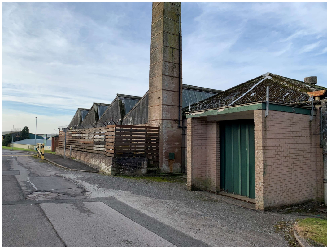
Photo Plate No. 09: Unoccupied former works with Tank beyond barbed wire fence in south west.
