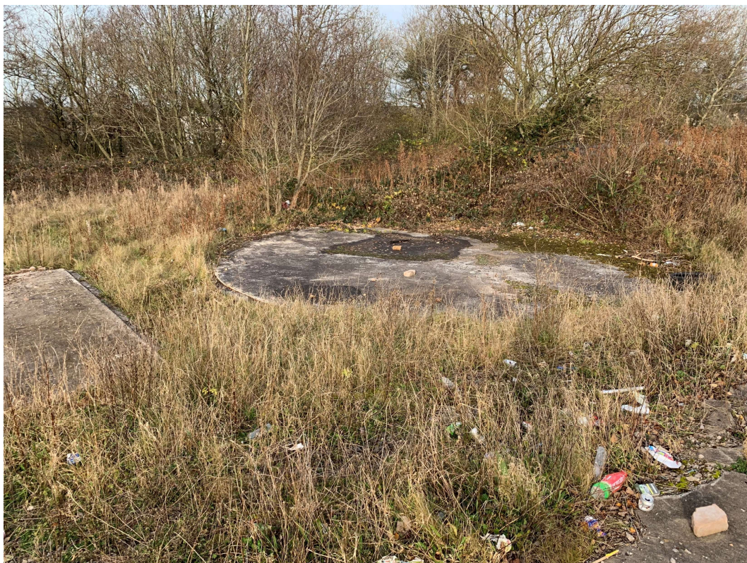
Photo Plate No. 11: Former tank pad in the west.
