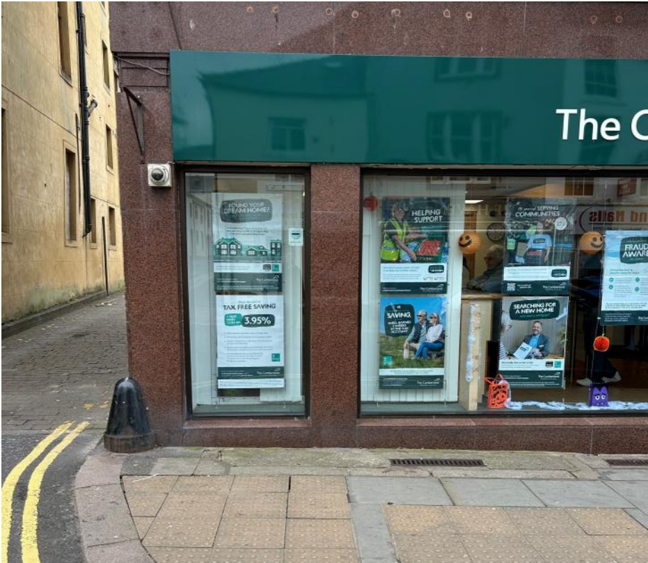
Image of Existing Façade at Ground Floor (left hand side)
