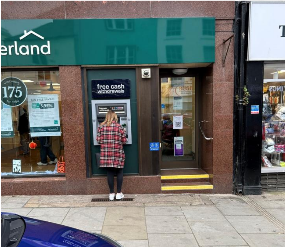
Image of Existing Façade at Ground Floor (right hand side)
