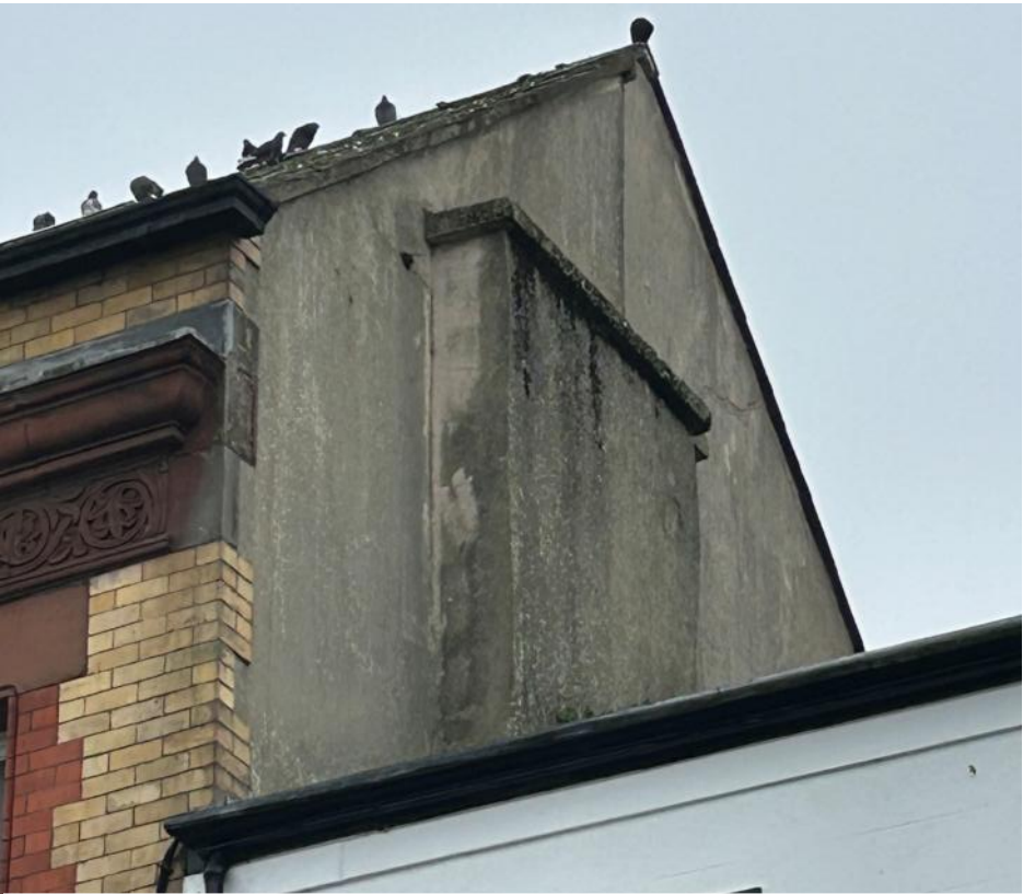
Picture of Building Above Neighbouring Property
