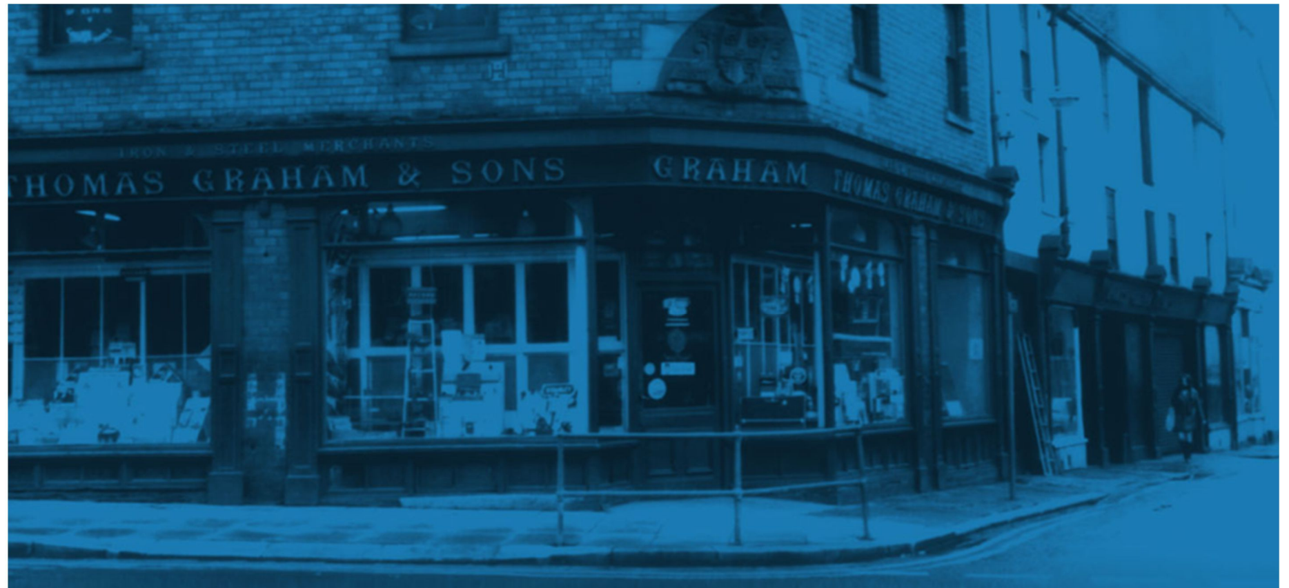
Figure 2: Thomas Graham’s ironmongery shop and steel warehouse , Lowther Street, Carlisle
