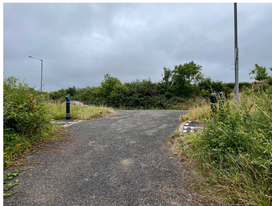
Figure 6: Looking out of site to existing access
