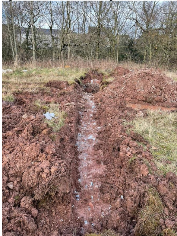
Figure 12: Area of slit trenching around Shaft 006.
