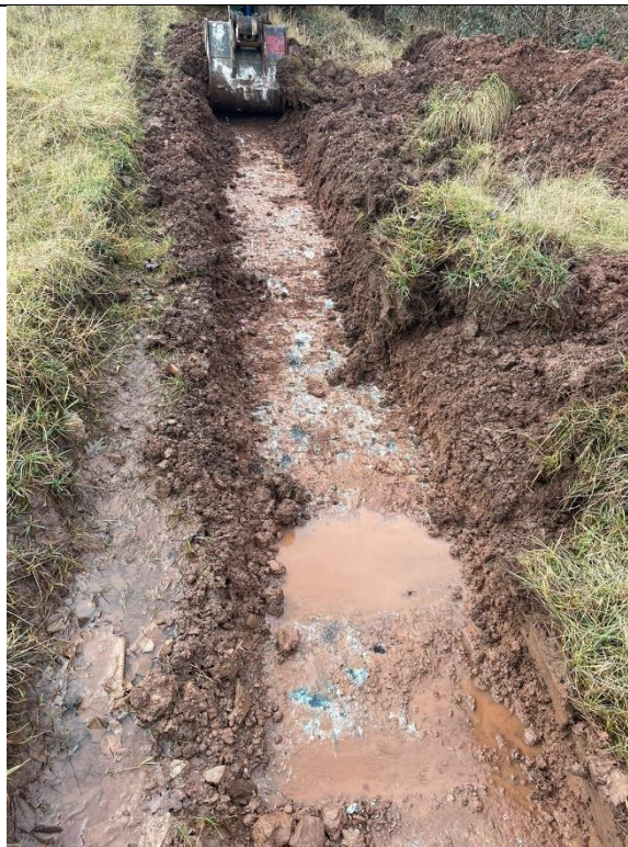
Figure 11: Area of slit trenching around Shaft 006.
