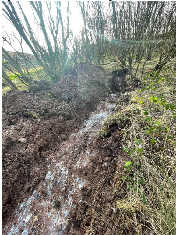
Figure 14: Area of slit trenching around Shaft 008.
