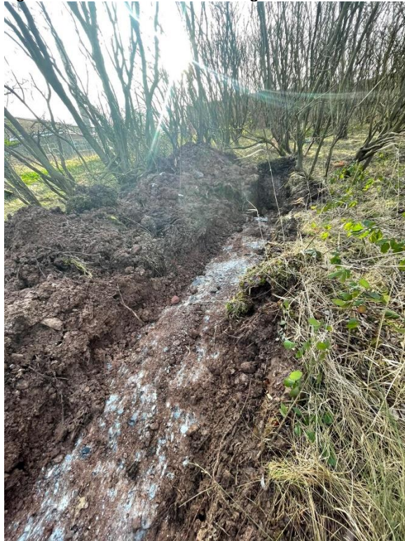
Figure 13: Area of slit trenching around Shaft 008.
