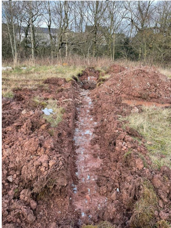
Figure 11: Area of slit trenching around Shaft 006.
