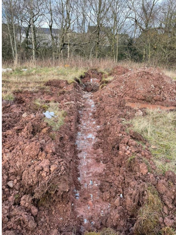
Figure 11: Area of slit trenching around Shaft 006.
