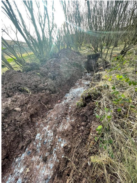
Figure 13: Area of slit trenching around Shaft 008.
