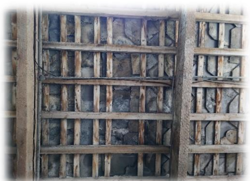
Plate 13: Interior extension roof.
