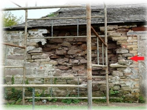
Plate 10: Exposed internal wall E aspect).
