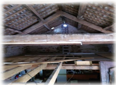
Plate 11: Barn 1 interior, showing removed timbers.
