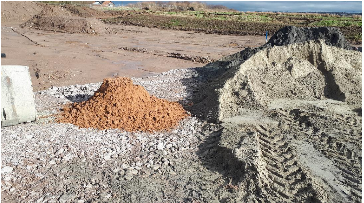
Photograph 9: Sand addition to grout mix.
