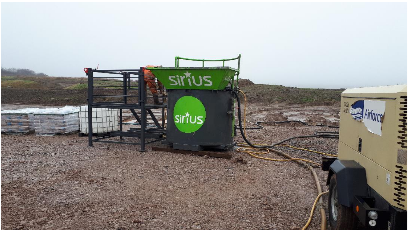
Photograph 3: Grout mixer, platform, compressor and OPC stockpile.
