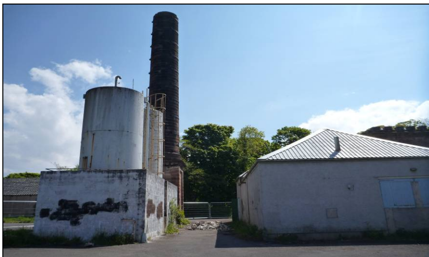
Photo 5: Chimney and oil tanks to north of the end of the southeastern end of the mill building, facing east
