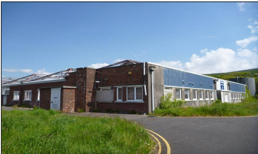
Photo 15: Gates factory to east of site, from west
