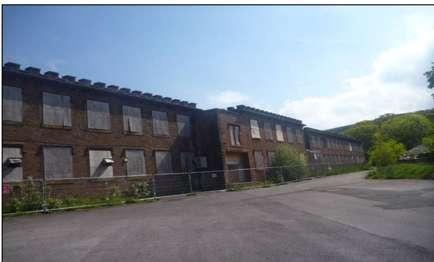
Photo 3: Southern end of old mill, in far south of the site, from Mill Street
