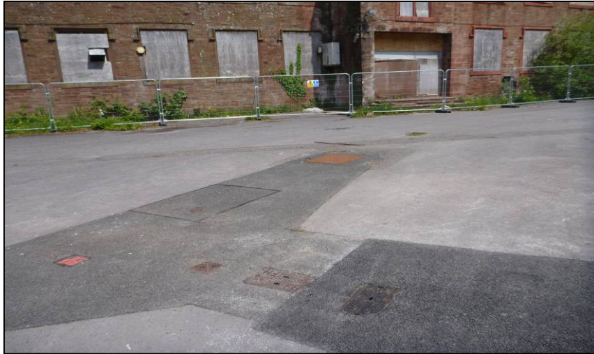
Photo 4: Probably original path of the mill race to the south
