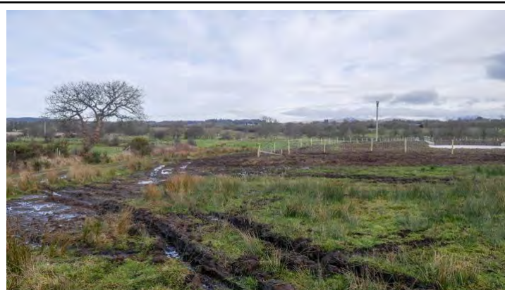
8. View of SUDS feature which serves Phase 1
