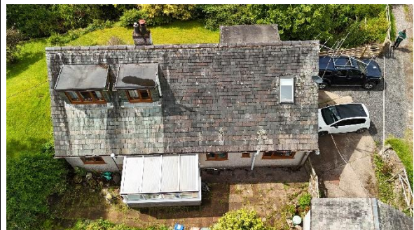
Photo 18: aerial view of eastern roof
