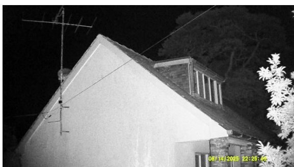
Photo 25: 14.08.25 S4 survey end, IR on
