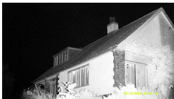
Photo 25: 14.08.25 S3 survey end, IR on
