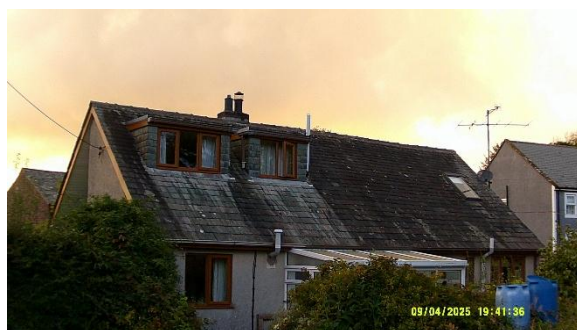
Photo 25: 04.09.25 S2 survey start
