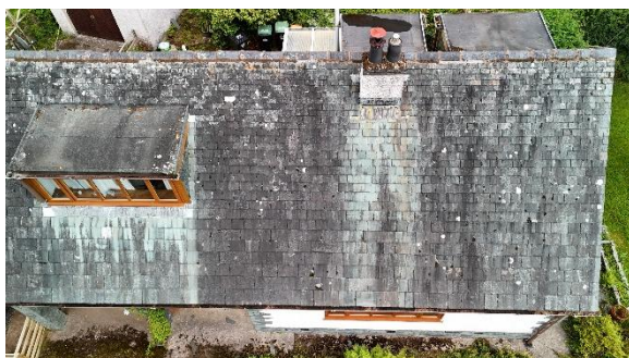
Photo 17: aera proposed for solar array
