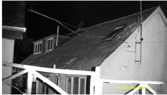
Photo 25: 14.08.25 S1 survey end, IR on
