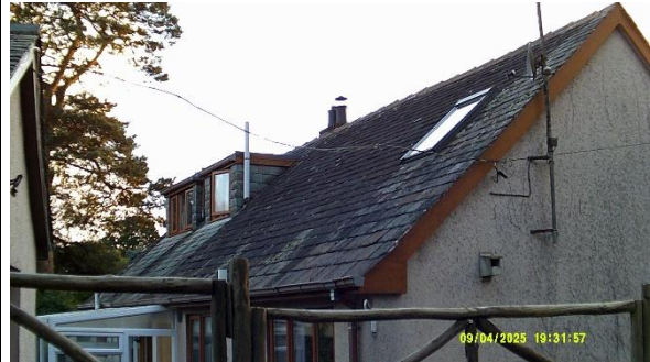
Photo 26: 04.09.25 S1 survey start
