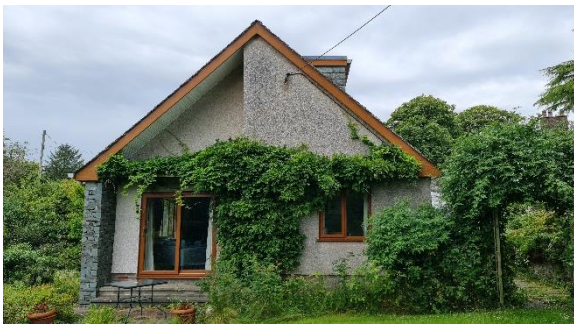
Photo 11: southern gable end
