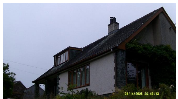
Photo 26: 14.08.25 S3 survey start
