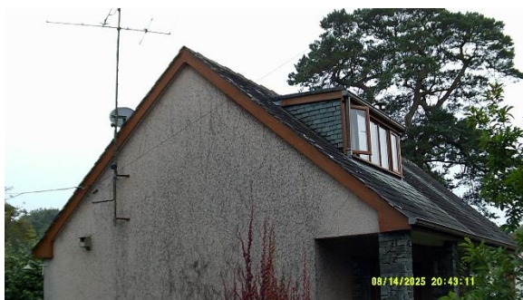
Photo 23: 14.08.25 S4 survey start
