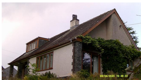
Photo 25: 04.09.25 S3 survey start
