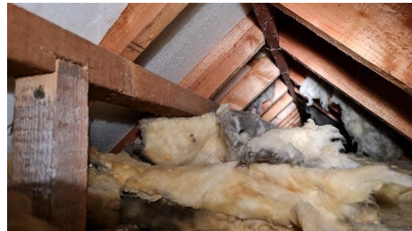
Photo 16: apex loft void
