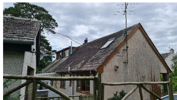
Photo 5: gable end and eastern roof
