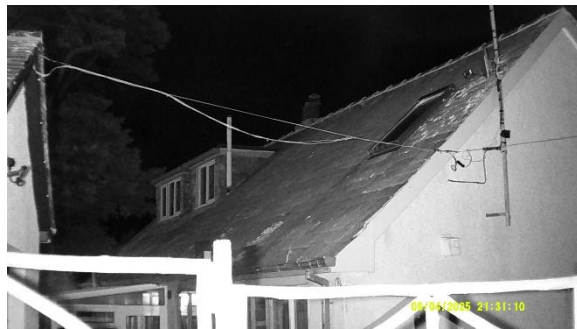
Photo 25: 04.09.25 S1 survey end, IR on
