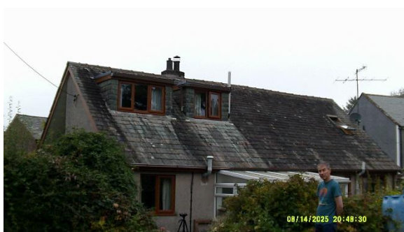
Photo 25: 14.08.25 S2 survey start
