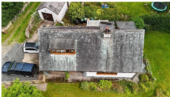
Photo 17: aerial view of western roof
