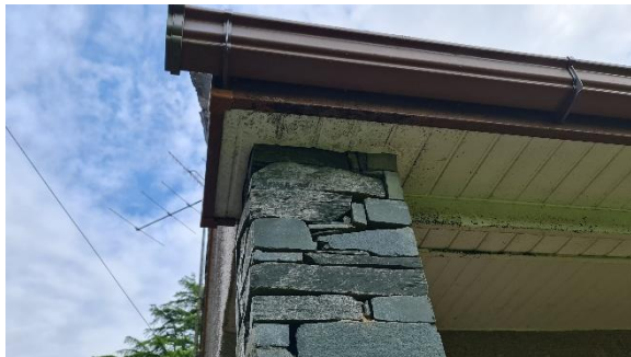
Photo 3: soffit and support pillar example
