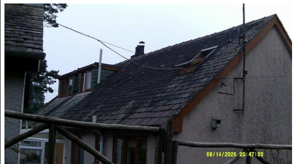
Photo 24: 14.08.25 S1 survey start
