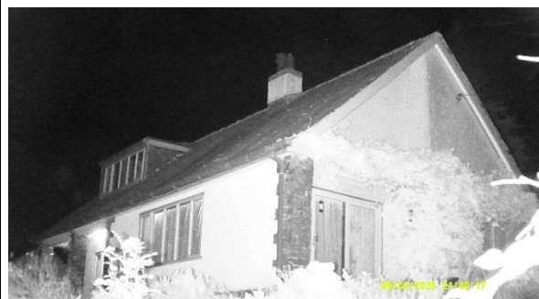
Photo 26: 04.09.25 S3 survey end, IR on
