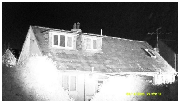
Photo 25: 14.08.25 S2 survey end, IR on
