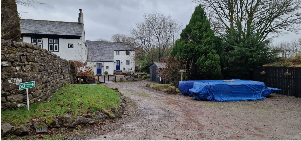
View from Car Park towards Old Hayloft with Shed behind Trees
