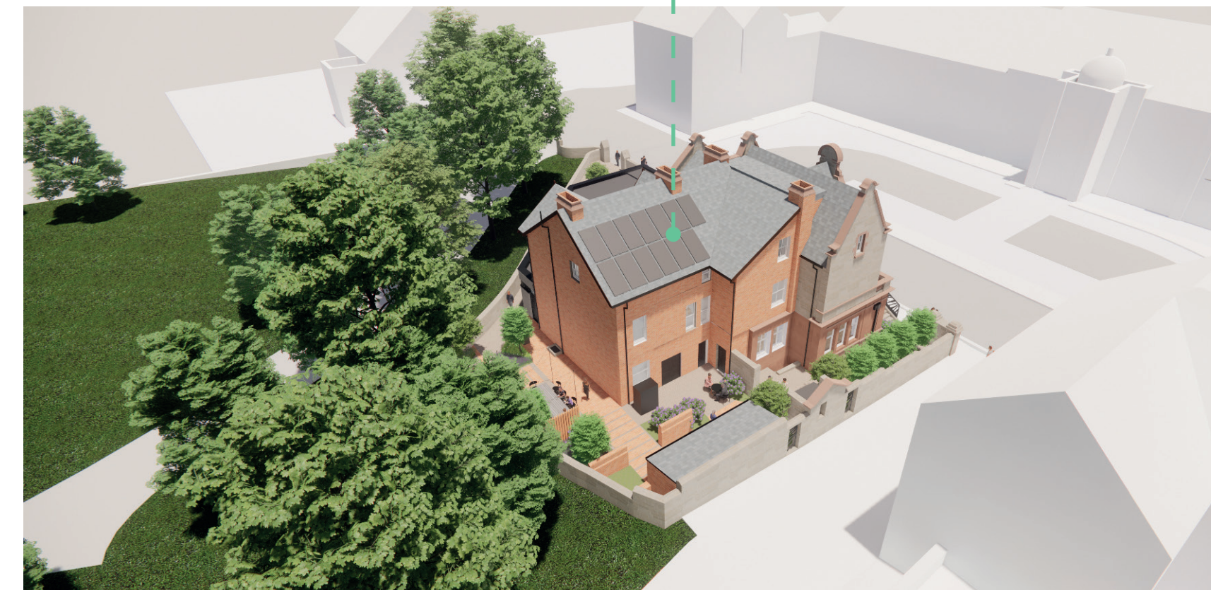
FIG 14 Refurbished Garden area and Photovoltaic Panles ro rear roof pitch.
