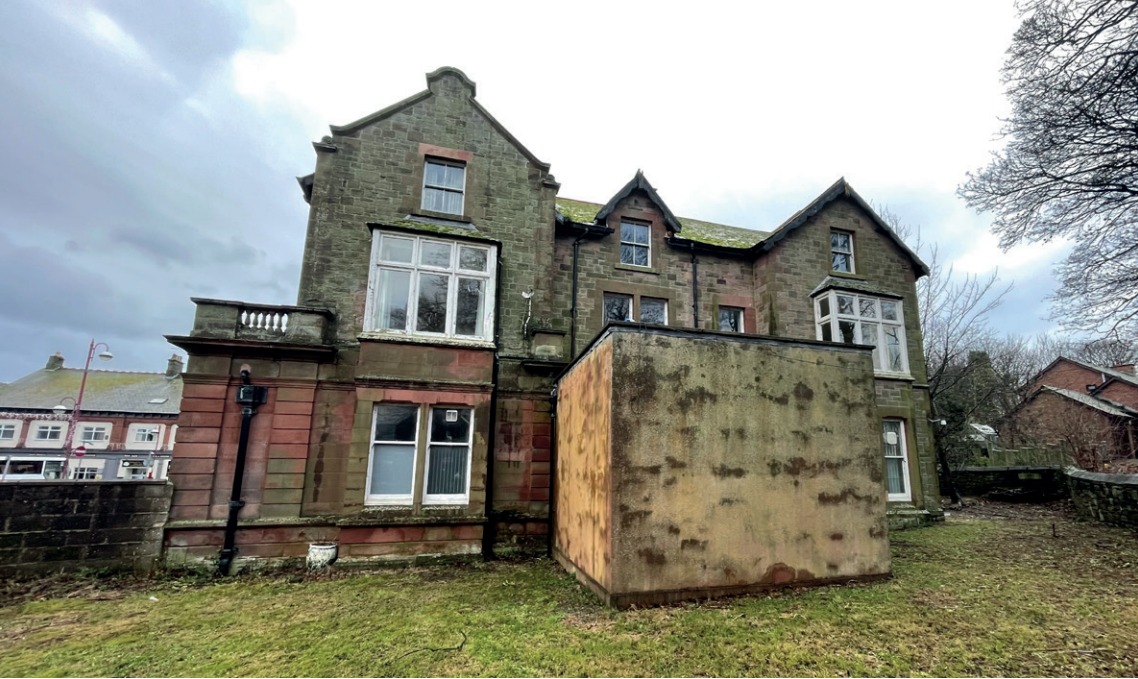
North West, Rear Elevation showing Bank Vault
