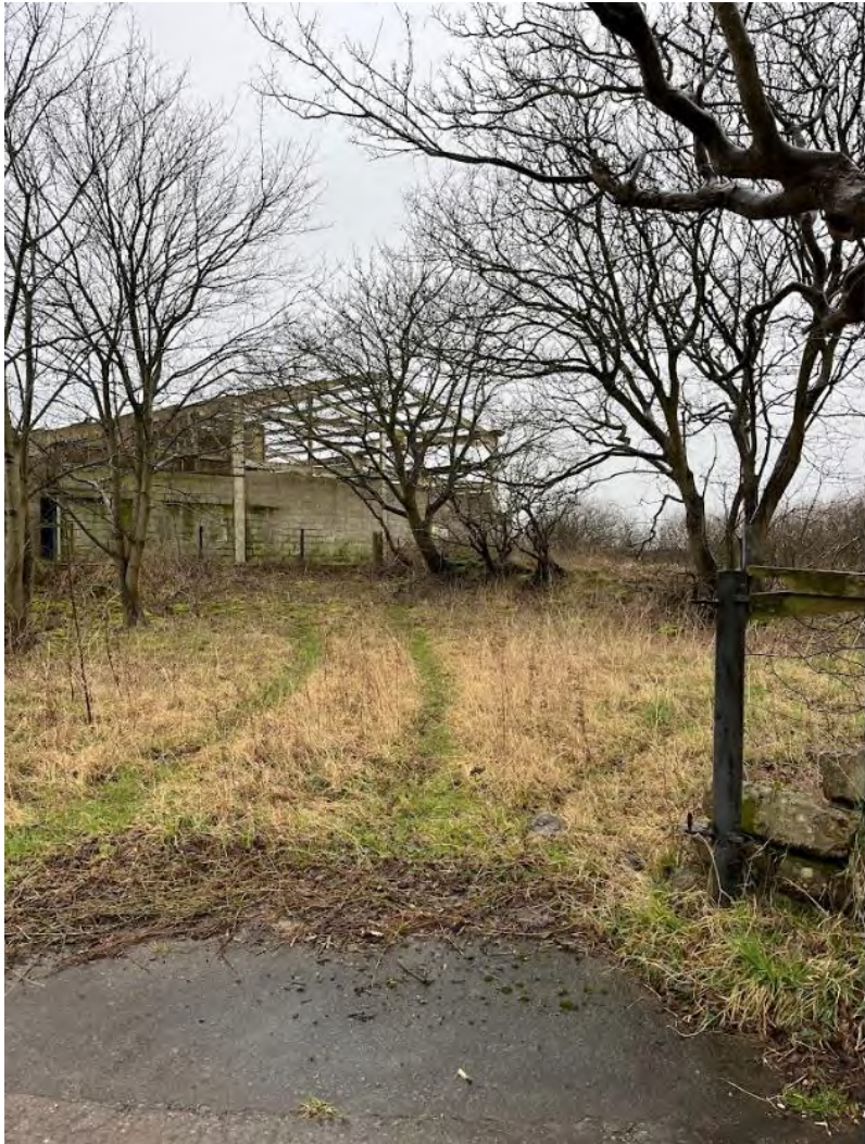
Figure 9 - Looking southeast towards largest site building.
