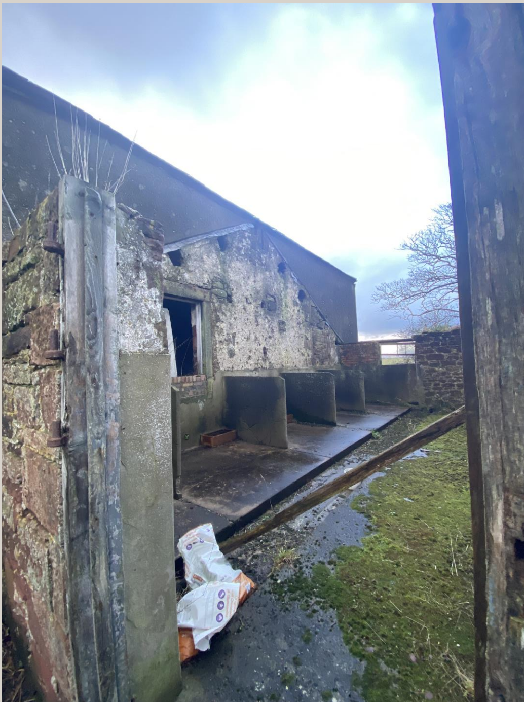
Photograph 6. Stone Building adjoining High House
