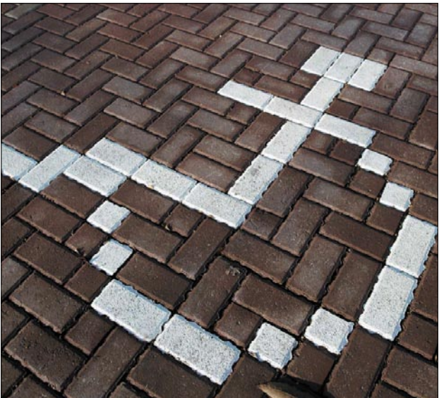
Colourtrop Priora, Martlesham Park & Ride, Ipswich used for marking out disabled parking bays
