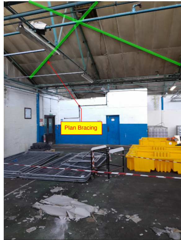
Figure 50 - existing buildings to be demolished , INTERNAL ROOF TRUSS, HALF HEIGHT MASONRY WALL
