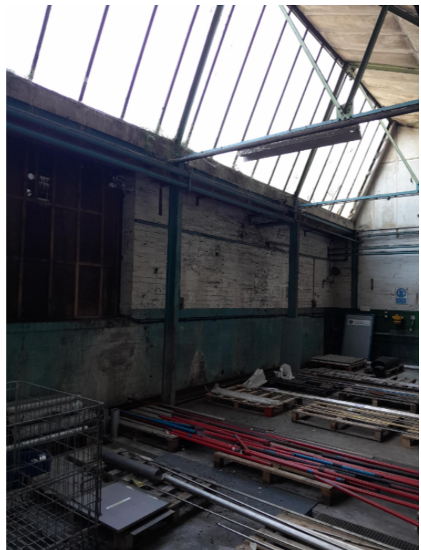
Figure 58 - INTERNAL SPINE WALL spans full height to valley gutter for the last TWO bays closest to SE elevation
