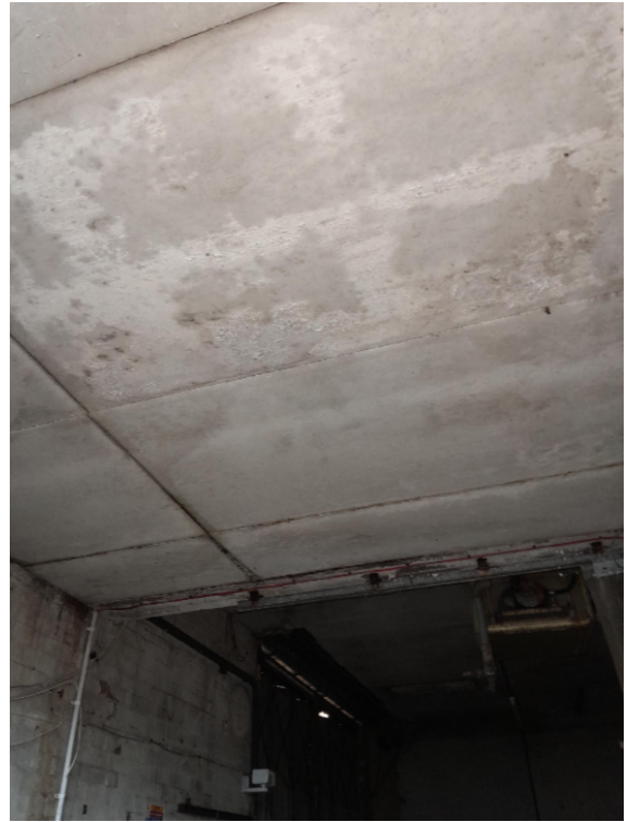
Figure 51 - existing buildings to be demolished , SCREWED ON SOFFIT, CONCRETE LINTEL
