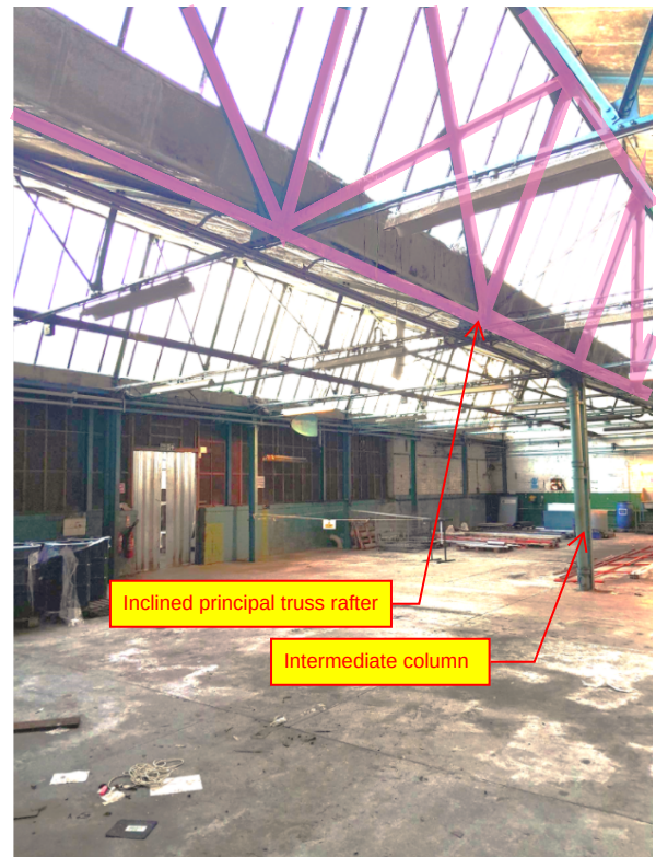
Figure 44 - existing buildings to be demolished , FLAT ROOF TRUSS adjacent to glazing
