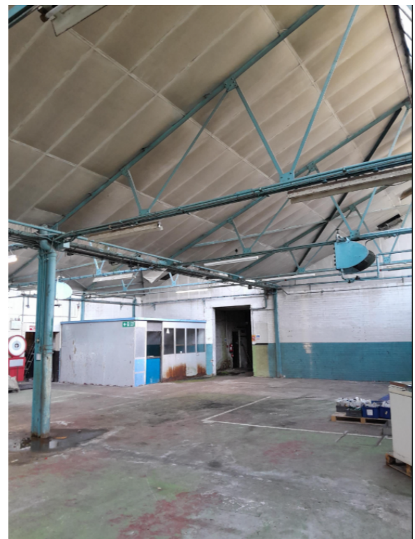
Figure 48 - existing buildings to be demolished , INTERNAL ROOF TRUSS, LGS free standing structure
