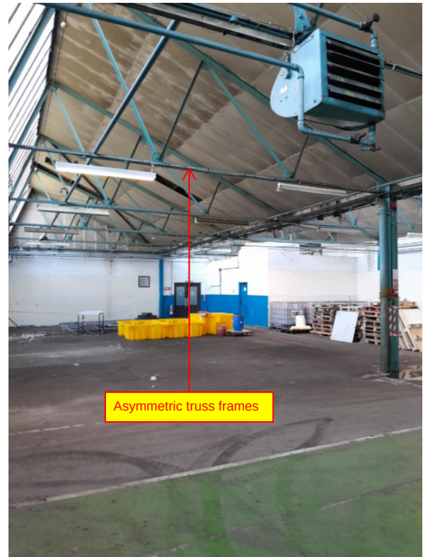
Figure 48 - existing buildings to be demolished , INTERNAL ROOF TRUSS, LGS free standing structure
