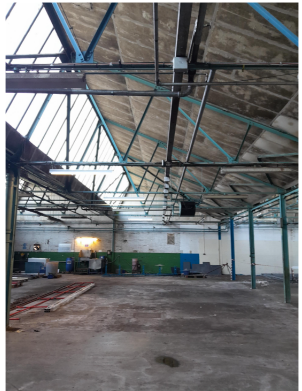
Figure 44 - existing buildings to be demolished , FLAT ROOF TRUSS adjacent to glazing
