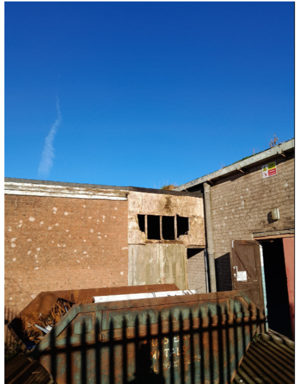
Figure 56 - existing buildings to be demolished , FLAT ROOF, TIMBER JOISTS, DIAGONAL CRACK
