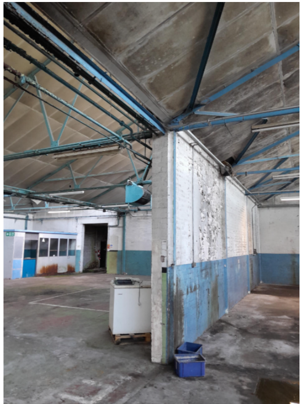
Figure 46 - existing buildings to be demolished , TWO-BRICK THICK MASONRY WALL
