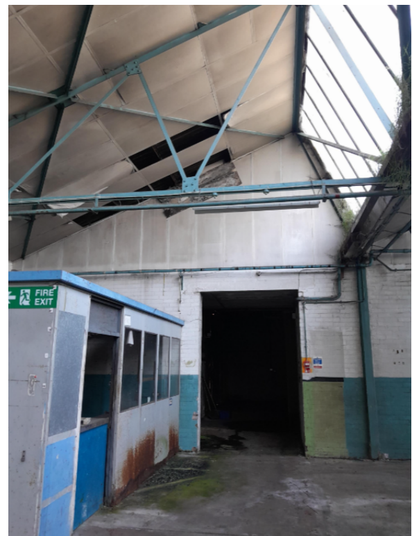
Figure 50 - existing buildings to be demolished , INTERNAL ROOF TRUSS, HALF HEIGHT MASONRY WALL
