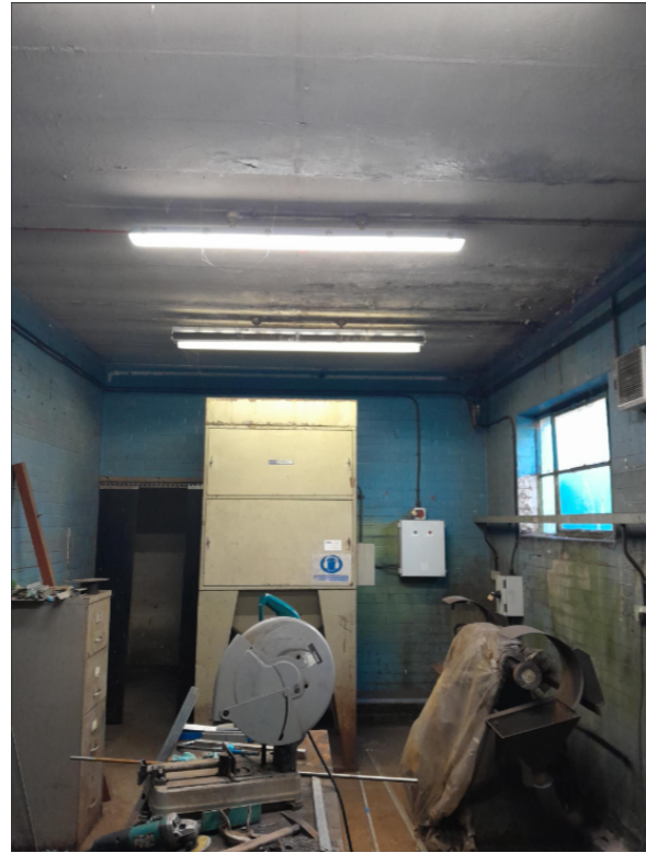
Figure 34 - existing buildings VIEW OF INTERNAL SPINE WALL which is to remain taken from retained side
