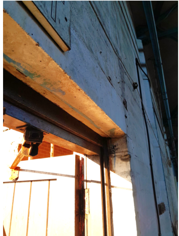
Figure 58 - INTERNAL SPINE WALL spans full height to valley gutter for the last TWO bays closest to SE elevation
