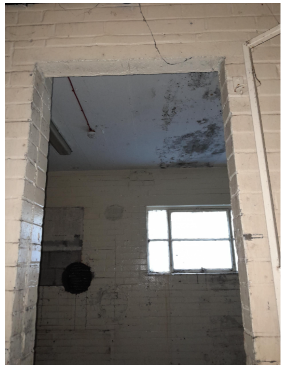
Figure 30 - existing buildings to be demolished , APPEARS AS CONCRETE SOFFIT to single storey. LB Masonry
