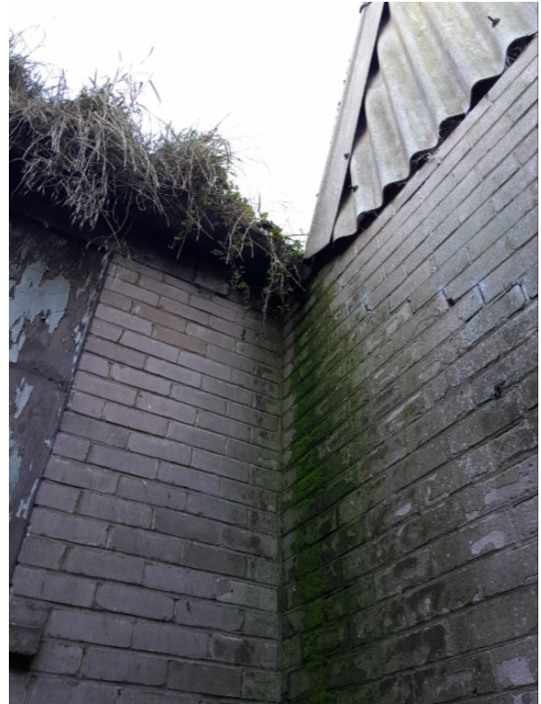
Figure 41 - internal spine wall and truss column (LEFT) to remain, perpendicular wall to be demolished
