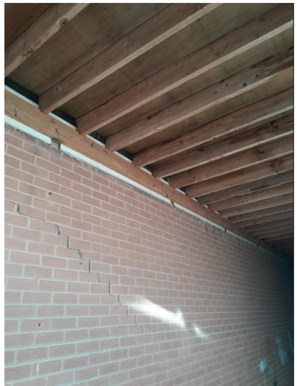
Figure 56 - existing buildings to be demolished , FLAT ROOF, TIMBER JOISTS, DIAGONAL CRACK
