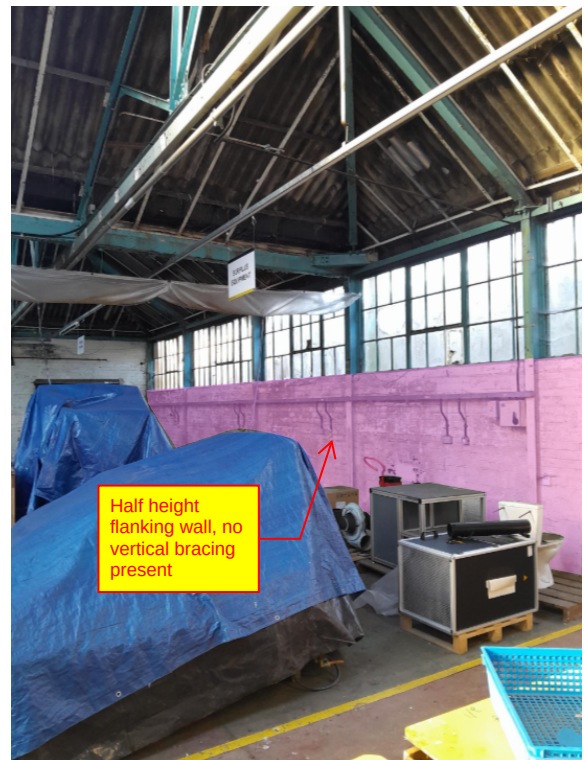
Figure 28 - existing buildings VIEW OF HALF-HEIGHT MASONRY WALL taken from retained side
