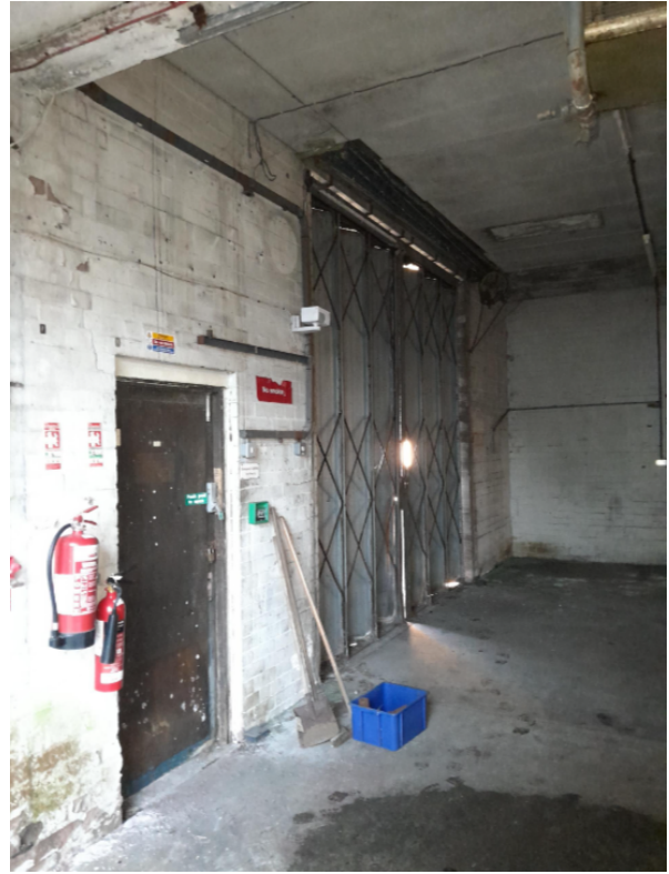
Figure 53 - existing buildings to be demolished , zone 3 internal view of ACCESS DOOR
