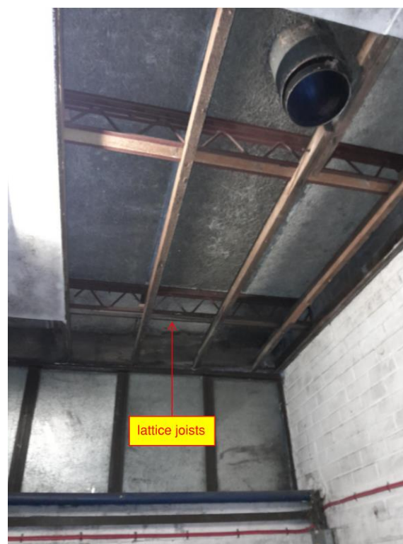
Figure 2.3 & Figure 2.4 – Zone 'C', single storey concrete slab soffit roof, load bearing masonry internal and external
