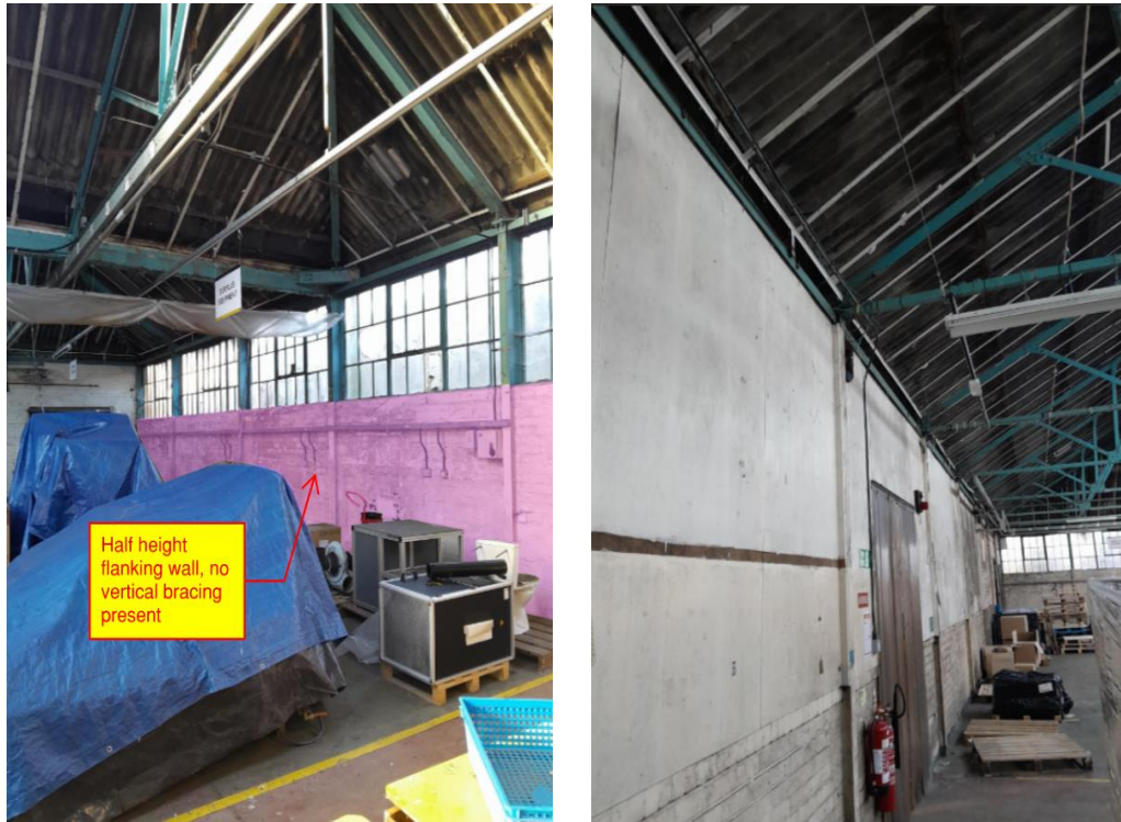
Figure 1.5 & Figure 1.6 – Zone 'A', half height flanking wall, and internal spine wall (right) to be retained
