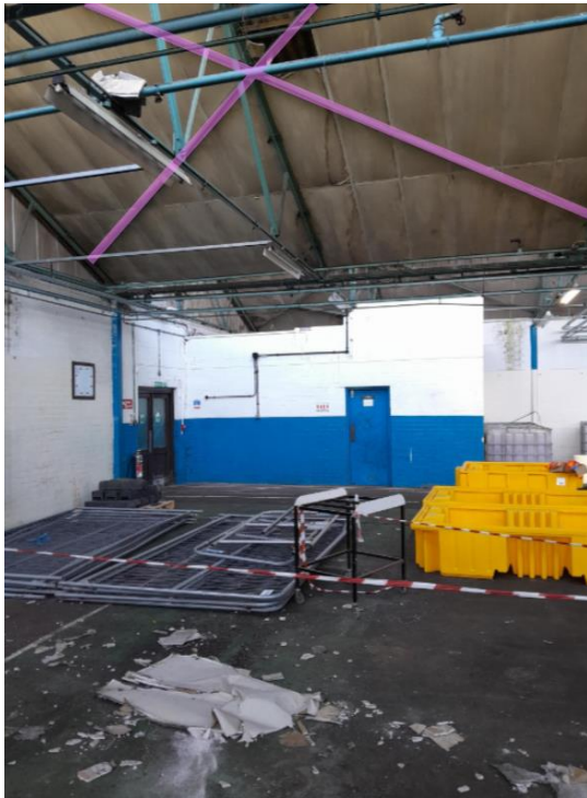
Figure 1.9 & Figure 2.0 – Zone 'B', main X-Angle bracing (left) and secondary K bracing (right)
