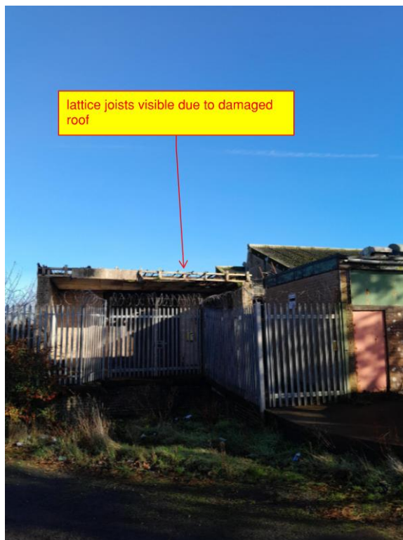
Figure 2.3 & Figure 2.4 – Zone 'C', single storey concrete slab soffit roof, load bearing masonry internal and external
