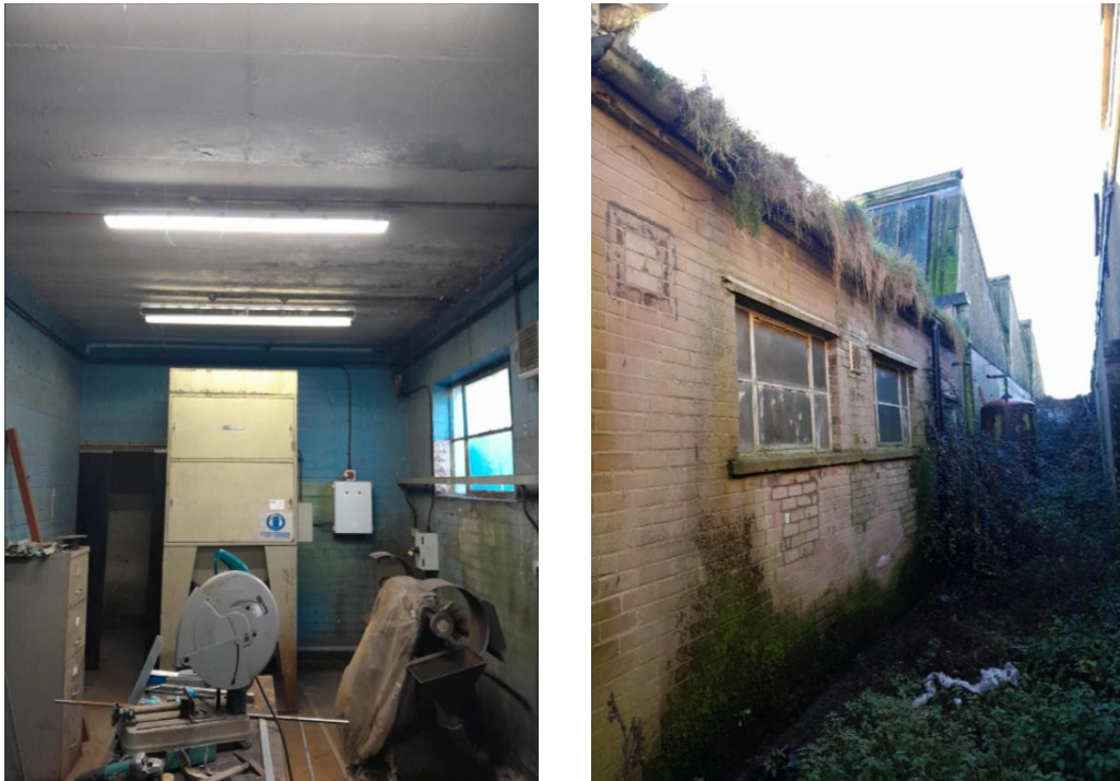
Figure 2.1 & Figure 2.2 – Zone 'C', single storey concrete slab soffit roof, load bearing masonry internal and external
