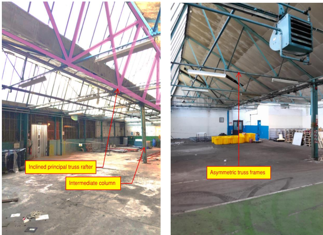
Figure 1.7 & Figure 1.8 – Zone 'B', principal truss rafter and asymmetric truss, roof construction
