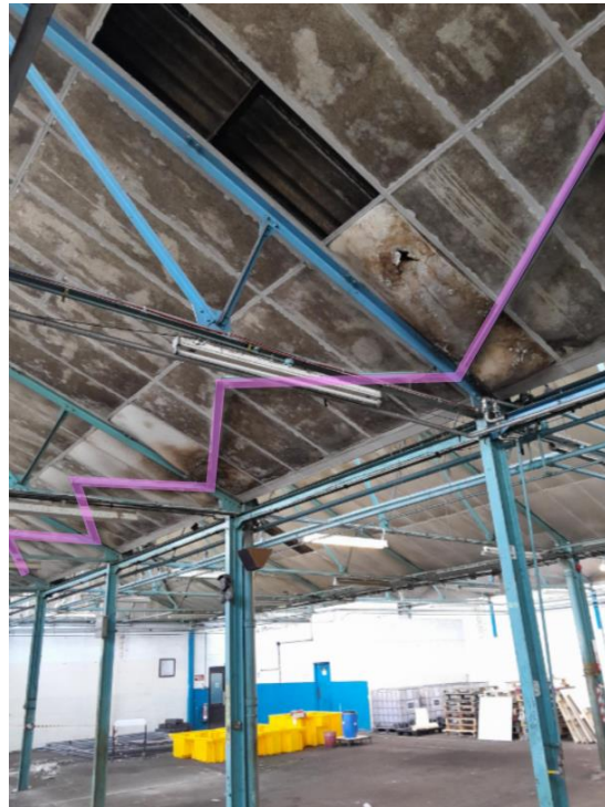
Figure 1.9 & Figure 2.0 – Zone 'B', main X-Angle bracing (left) and secondary K bracing (right)
