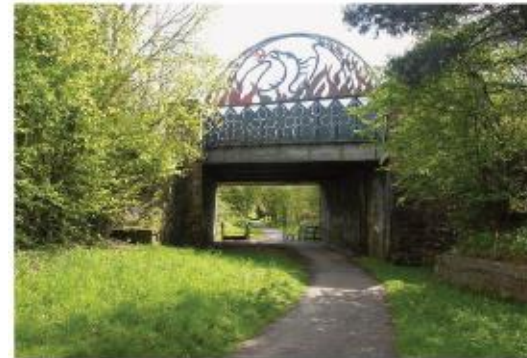
C2C Phoenix Bridge
