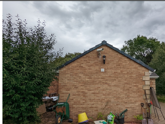
Photograph 2: North-western gable elevations
