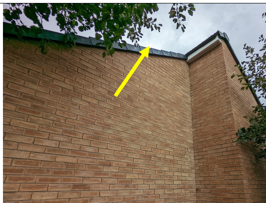
Photograph 3: North-eastern elevations, showing roost entry point
