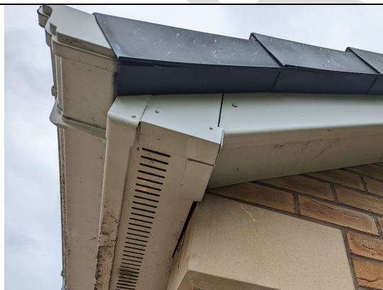
Photograph 5: Sealed soffit boxes
