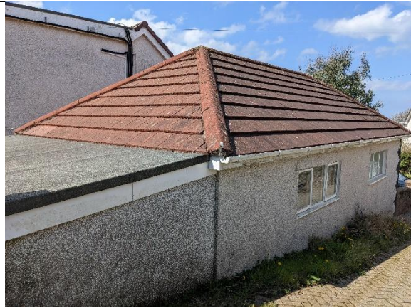
Photograph 1: Garage to be demolished
