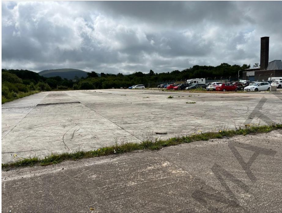
Photo 1: Photo taken looking southeast across area of hardstanding in west of the site.
