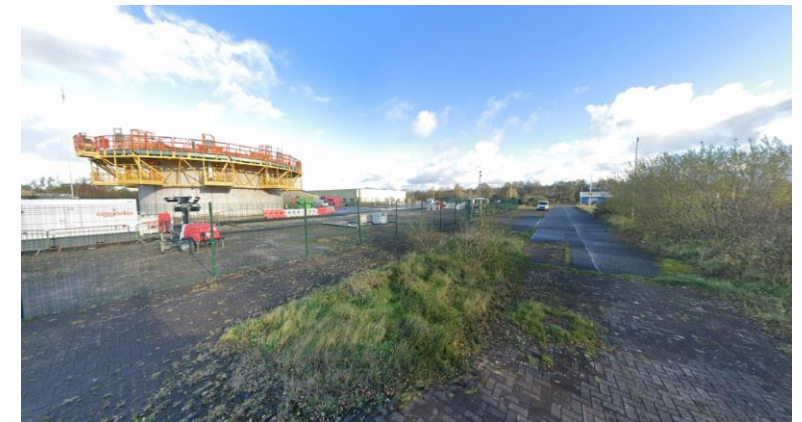
5. SPIDA site in the process of being demolished.
