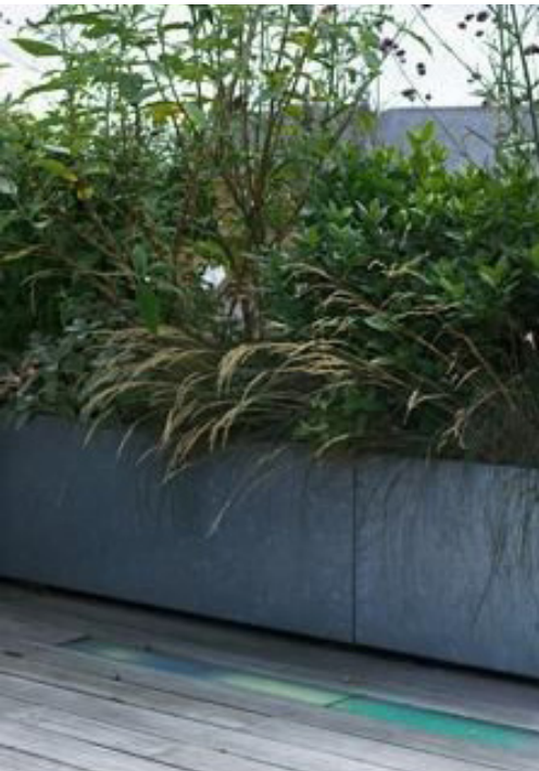
Precast concrete planters against wal Depth of planters 450mm Height of planters 600mm
