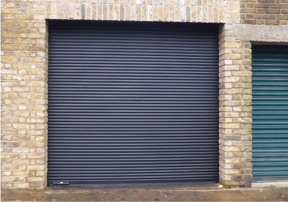
CGT Security Xonar 610 Security Shutter Concealed side guide cavity closers Powder coated finish colour matched to facade
