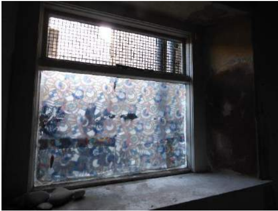
Left: The ground floor window to the rear is not original and requires repair / replacement subject to planning condition.
