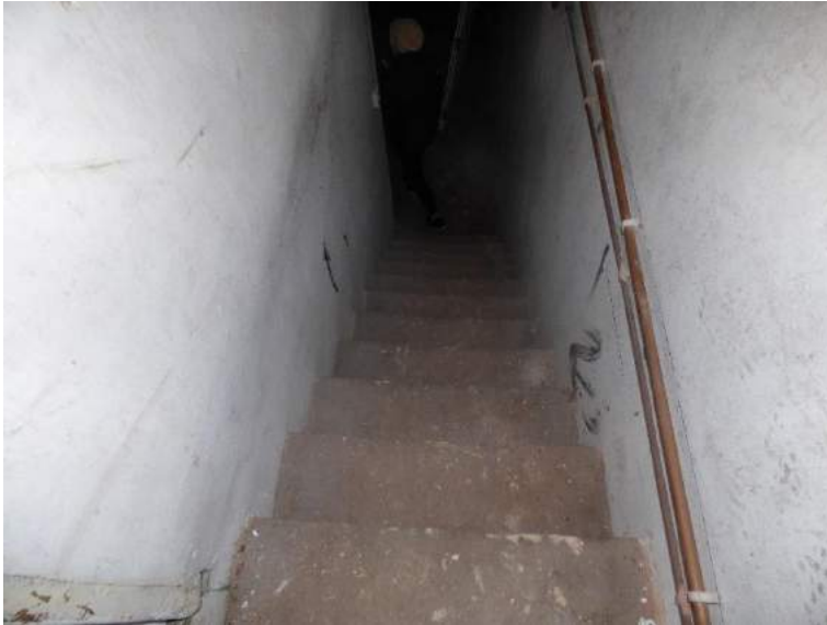
Left: The basement
