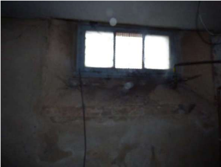
Existing window to basement to be repaired / replaced subject to planning condition.
