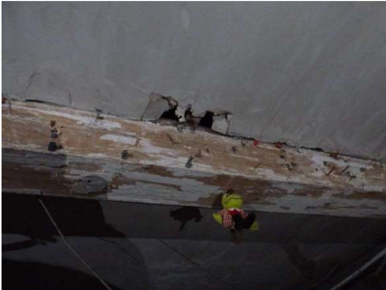
Left: Repairs to Fireline board or reinstatement to ensure fire resistance required to basement.
