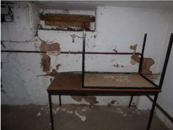
Left: The basement
