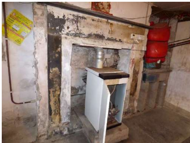
Left and above: Basement.
