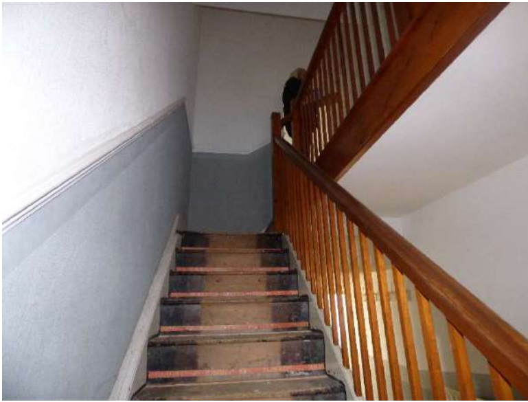
Left Retain staircase, which although not original is in good condition. Its is proposed to redecorate.
