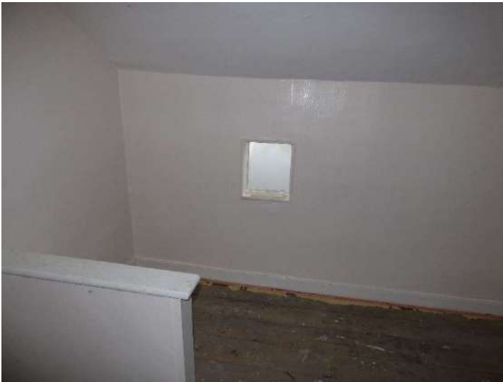
Left: Attic landing.
