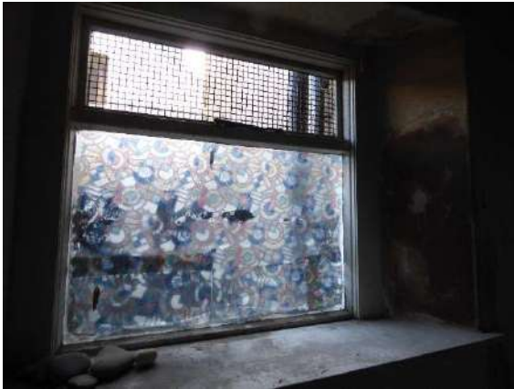
Left: The ground floor window to the rear is not original and requires replacement.
