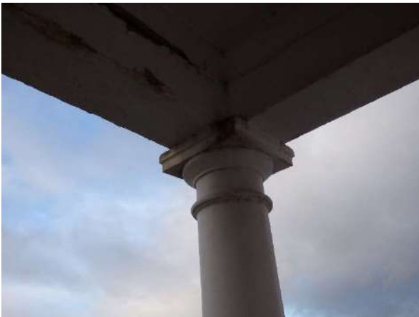
Left: Existing door to be repaired and rehung. Existing portico to be fully repaired and pillars to have paint removed and original stone restored.
