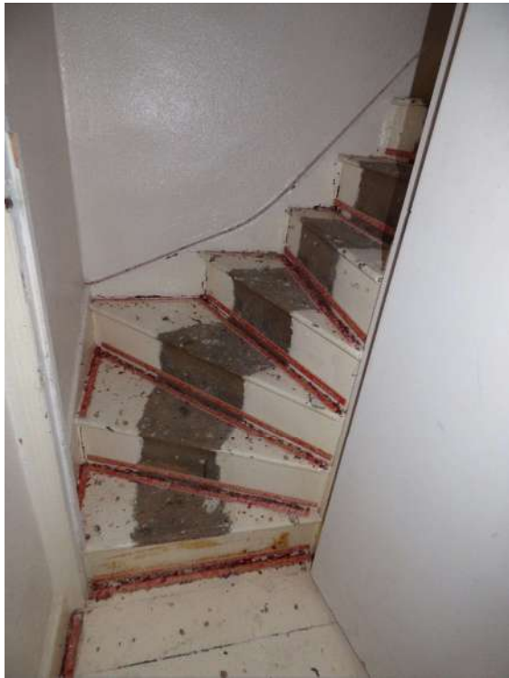
Above and right: Staircase to attic room.
