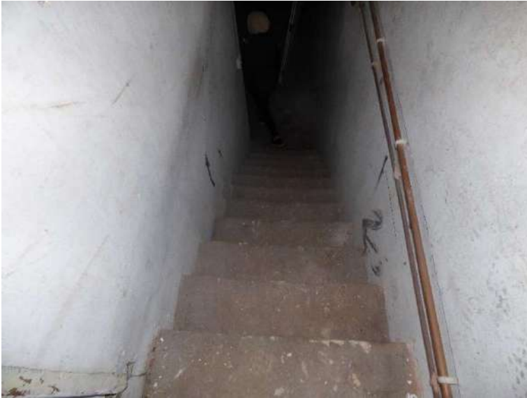
Left: The basement
