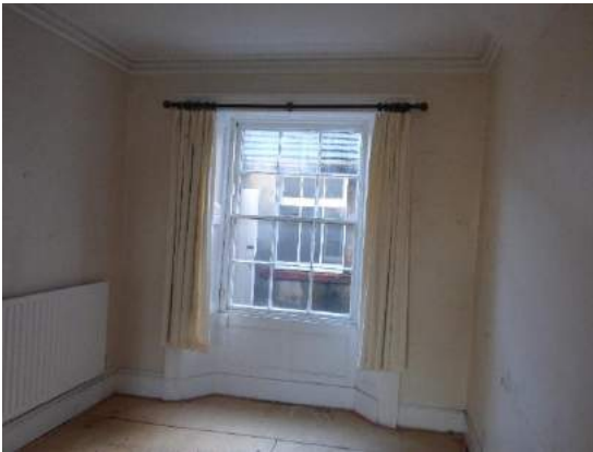
Above: Existing architraves, and skirtings to be retained and made good
