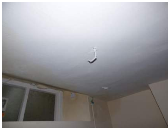
Views of existing basement.
