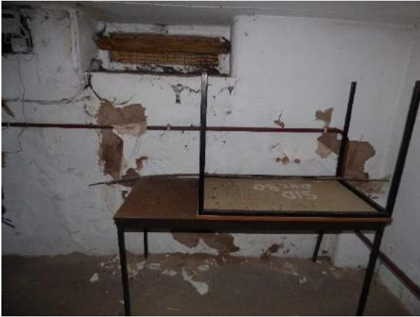
Left: The basement
