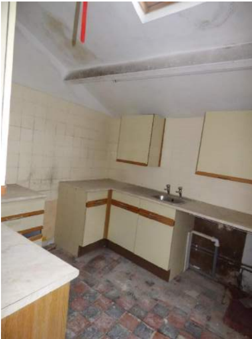
Left: Existing utility spaces to be fully renovated.
