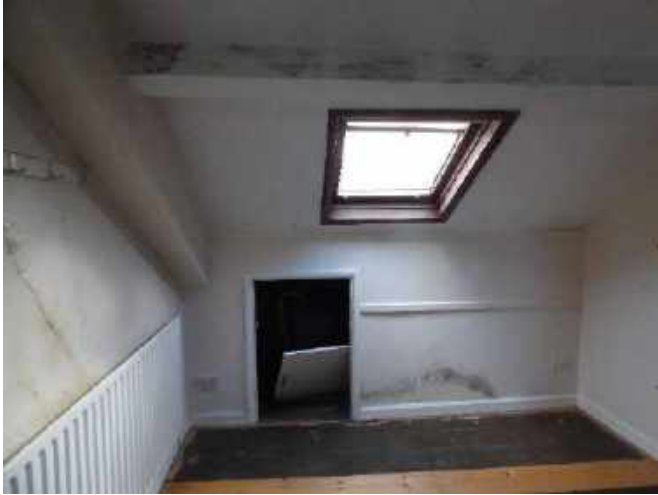
Left: Attic Bedroom
