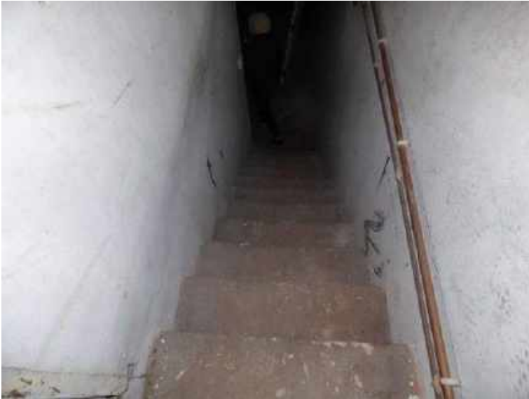
Left: The basement
