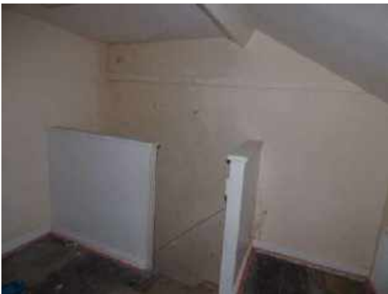
Left and below: Landing at the top of the staircase.
