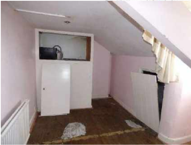
Left: Attic bedroom
