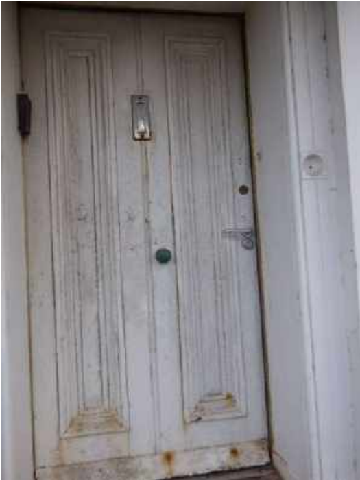
Left: Existing door to be repaired and rehung. Existing portico to be fully repaired and redecorated.
