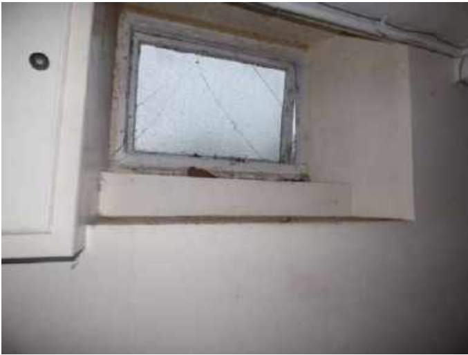
Left: Existing window to be replaced.
