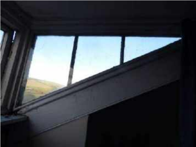
Left - Attic bedroom:
