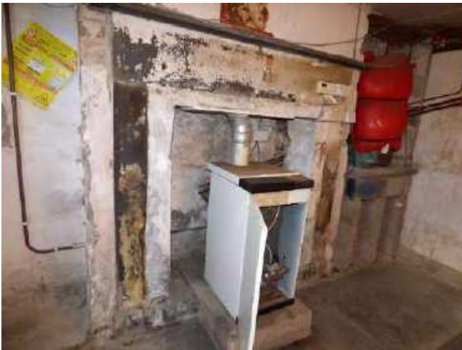
Left and above: Basement.
