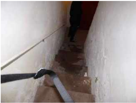
Left: The basement
