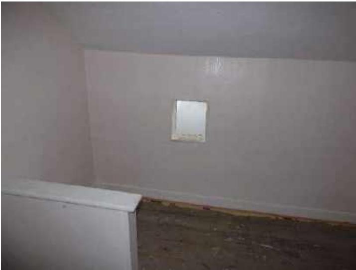
Left: Attic landing.
