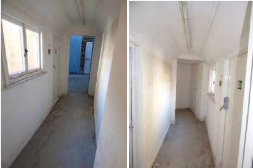
Left: Existing single skin ink building extension to be removed.
