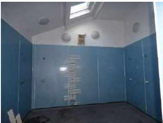
Left: original shower block to be reduced in size to provide additional amenity space to the property. All existing fixtures and fittings to be removed. The building then will become a new home office / store.
