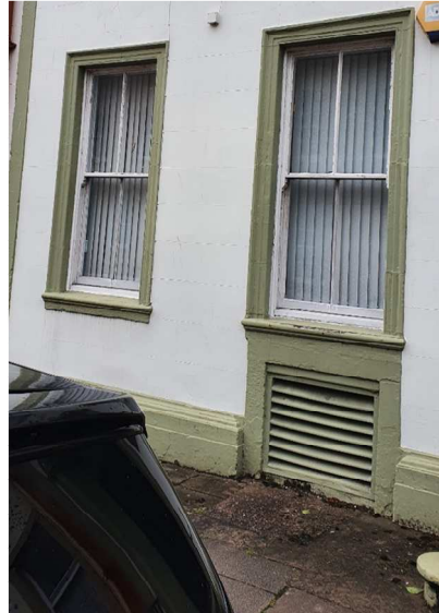
Traditional timber sash window with modern M&E louvre to basement.
