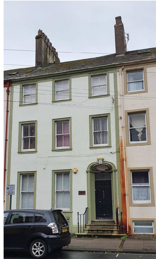
Listed Façade to be restored to original appearance with removal of louvre.
