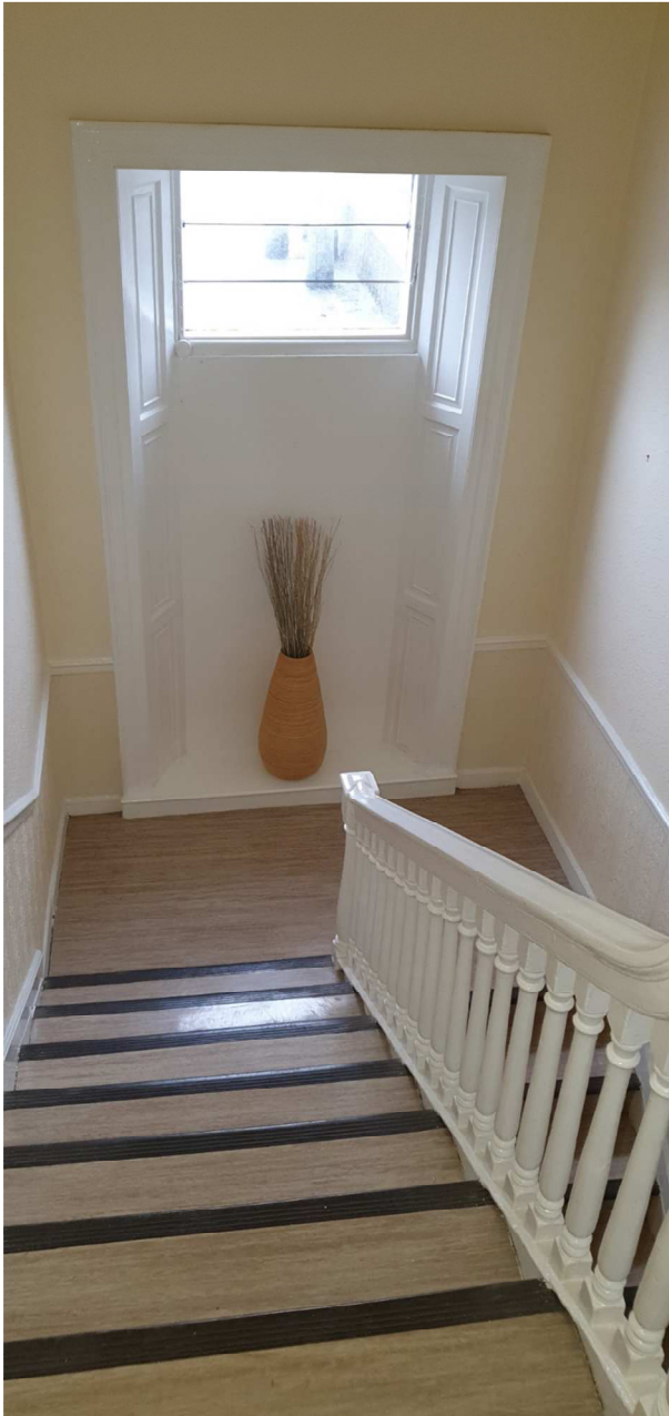
Original stair balustrade and splayed timber mouldings around windows.
