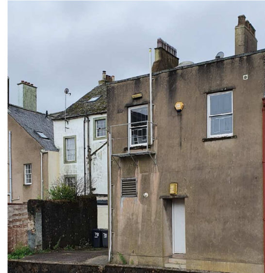
John's Lane Rear Elevation with redundant M&E Equipment and roughcast render.
