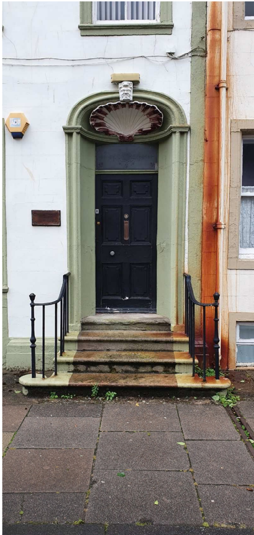
Traditional Georgian panel door, stone steps With architectural ironmongery and elliptical fanlight with decorative detail above door.
