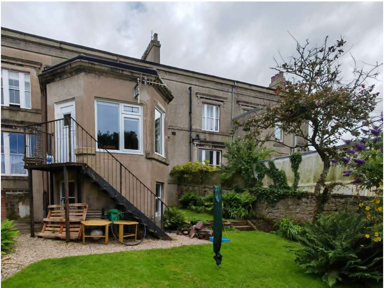
Photo 1- View of previous metal stair accessed from existing kitchen door
