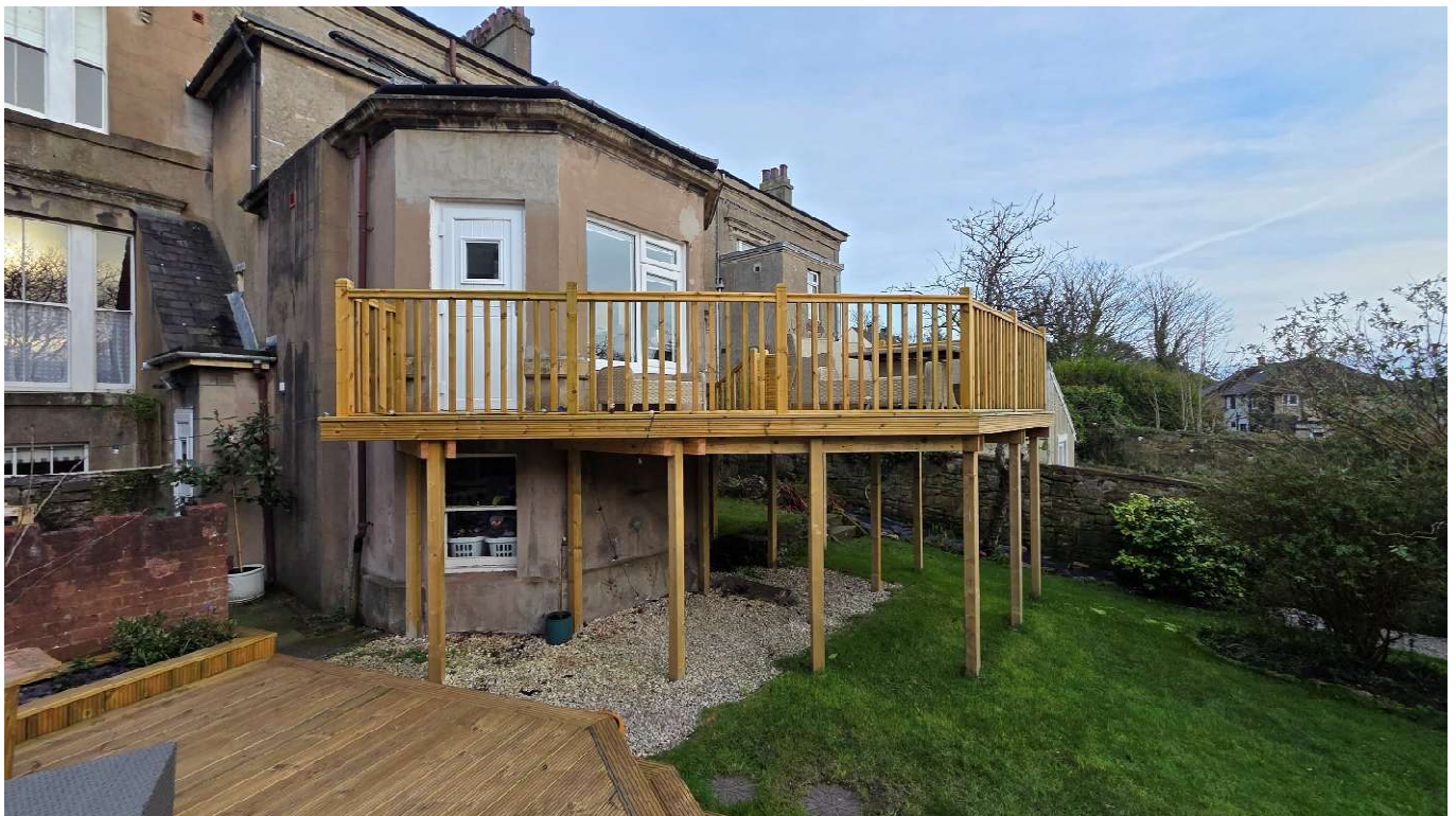
Photo 2 -Timber balcony as built
