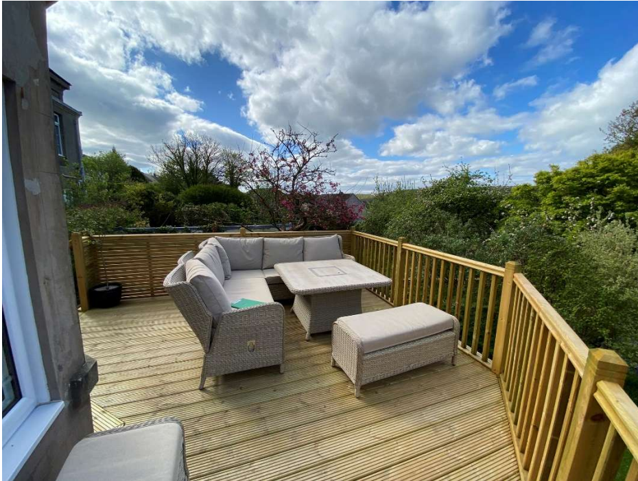
Photo 5 -Balcony as viewed from west side
