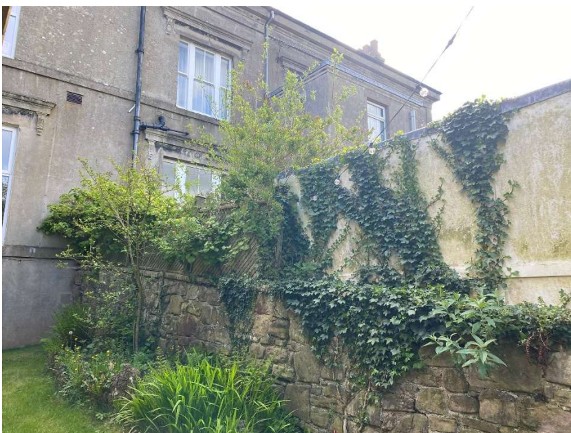
Photo 4 -Existing screening to neighbouring property
