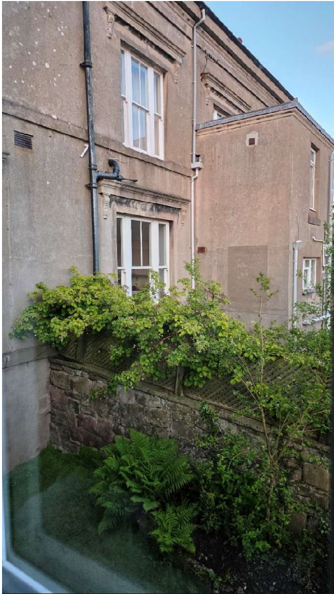
Photo 3 -Existing view to neighbour from kitchen window
