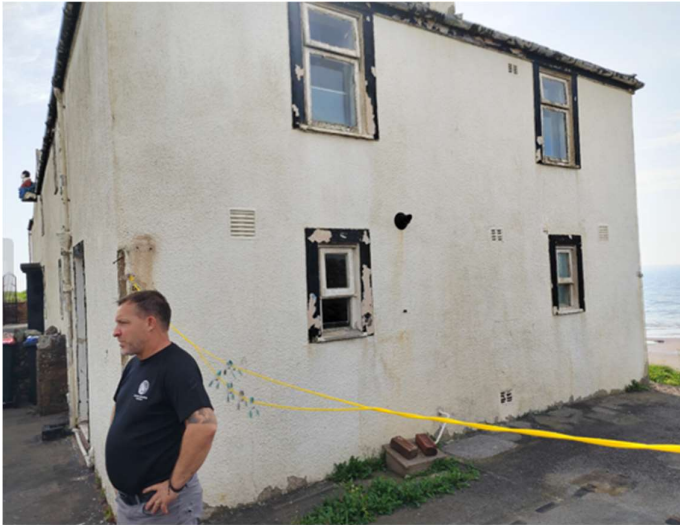
Side elevation of the property.
