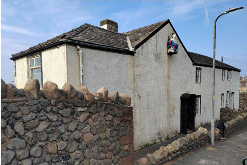
Front / Road elevation of the building
