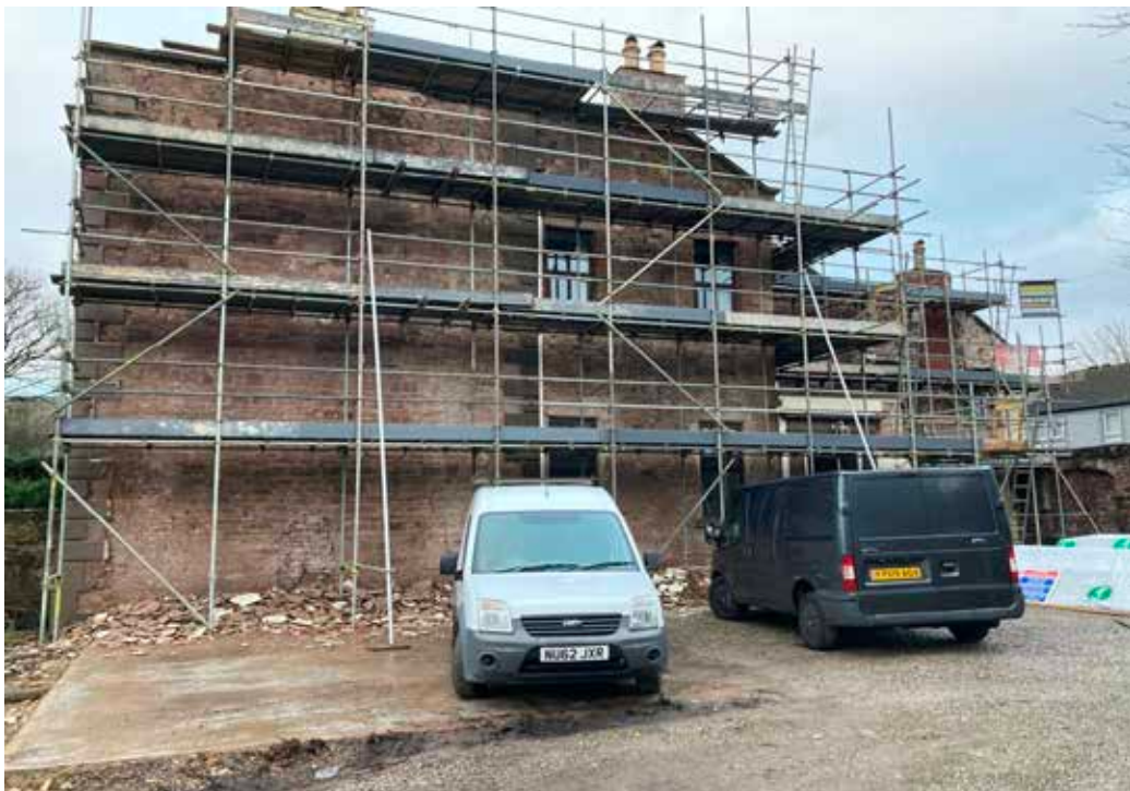
Photo 2: South elevation of Hensingham House.
