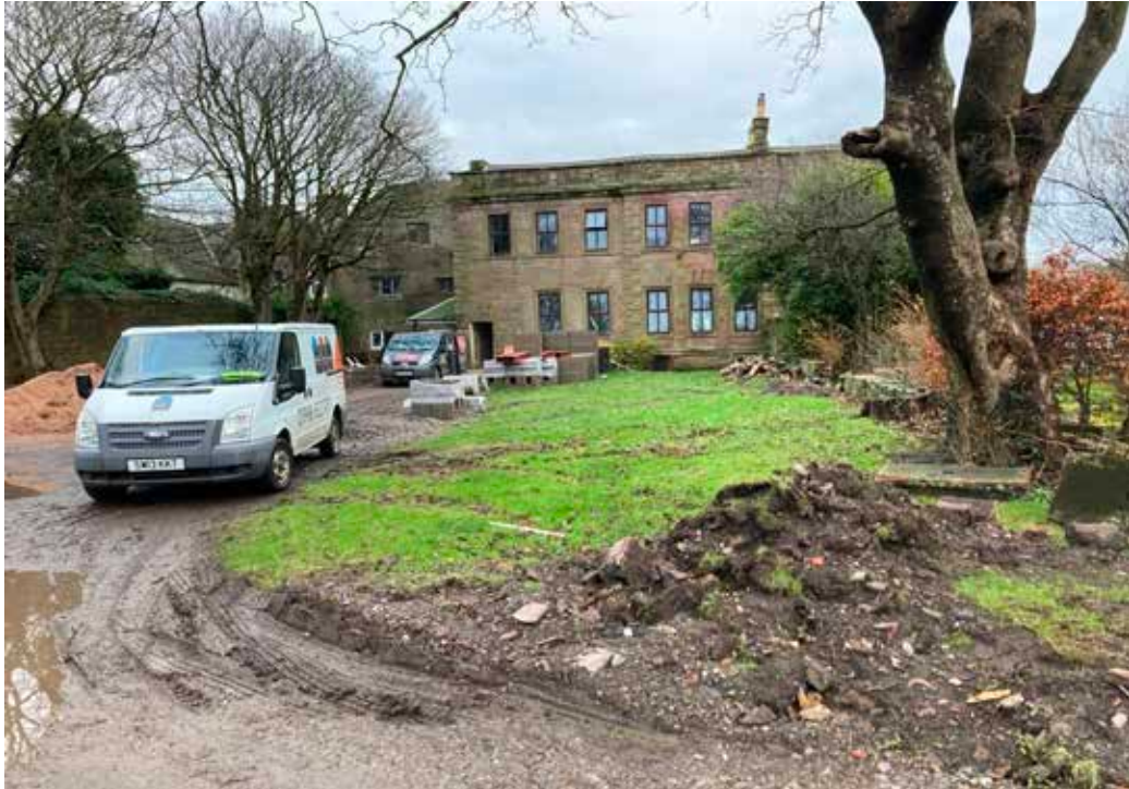
Photo 3: West elevation of Hensingham Hall. (Hensingham House obscured by tree on right).
