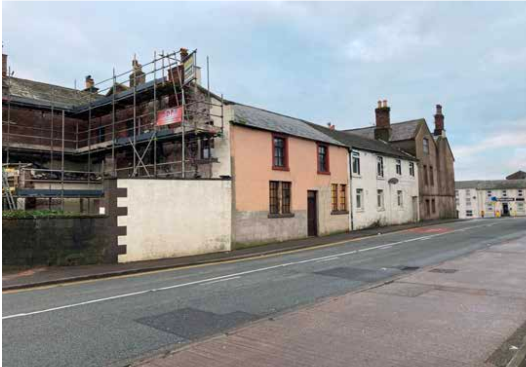
Photo 5: East elevation along Egremont Road.
