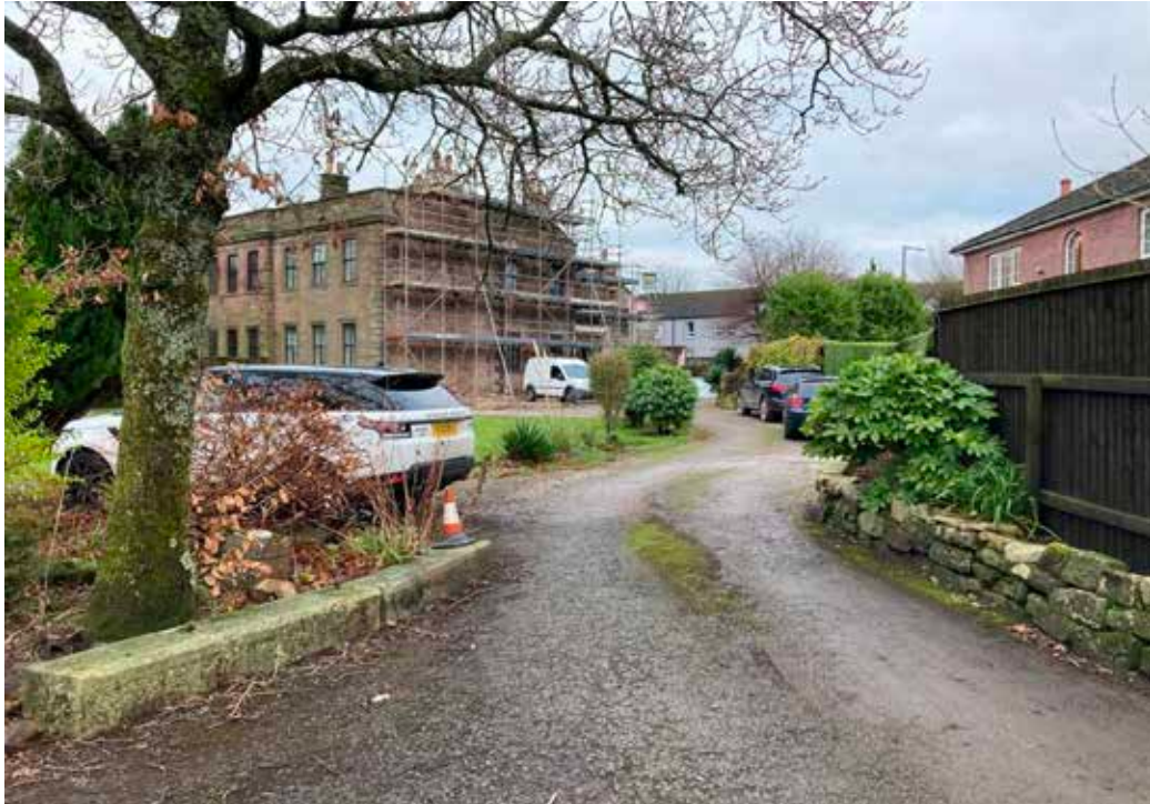
Photo 1: View from access road looking towards south elevation.
