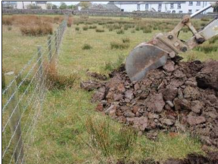
Photo 10: TP3 located on the south west of the site. The trial pit trenches were dug on both sides of the fence.
