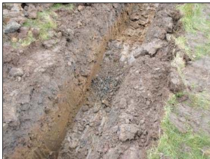
Photo 6: TP1 exposed gravel indicating a field drain location below.
