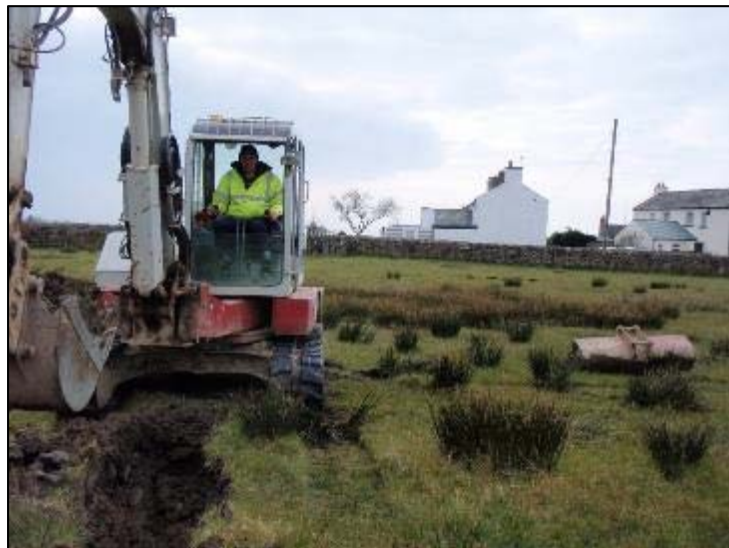
Photo 11: TP4 located in the south of the site.
