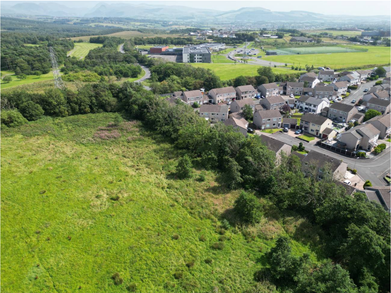
5 Group G3 at the southern boundary of the east section of the site.
