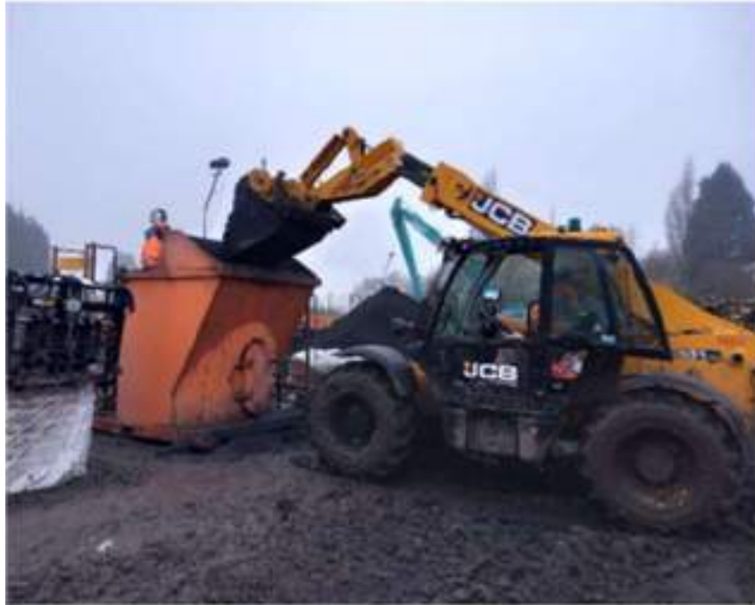
Figure 10: Grout mixer being loading by telehandler.
