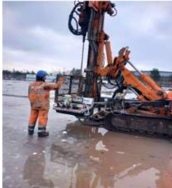
Figure 8: Checking mast is at the correct orientation.
