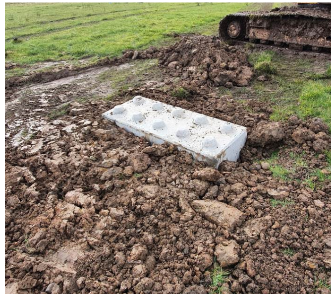
Figure 2: Arisings backfilled around blocks.
