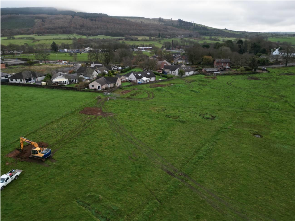
4. View of the southern boundary and proposed site access at Flosch Meadows.
