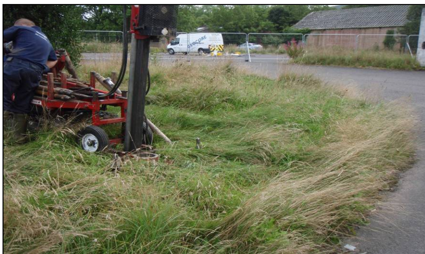
Photo 6: WS4 during drilling, on roundabout in the central area
