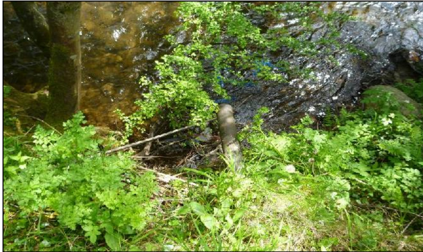
Photo 13: Outlet pipe to river from eastern section of the site
