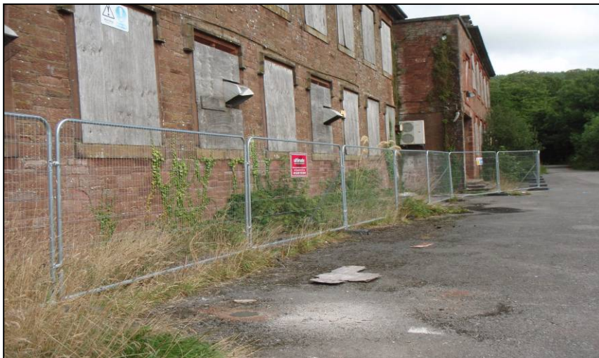
Photo 15: WS9 after backfilling
