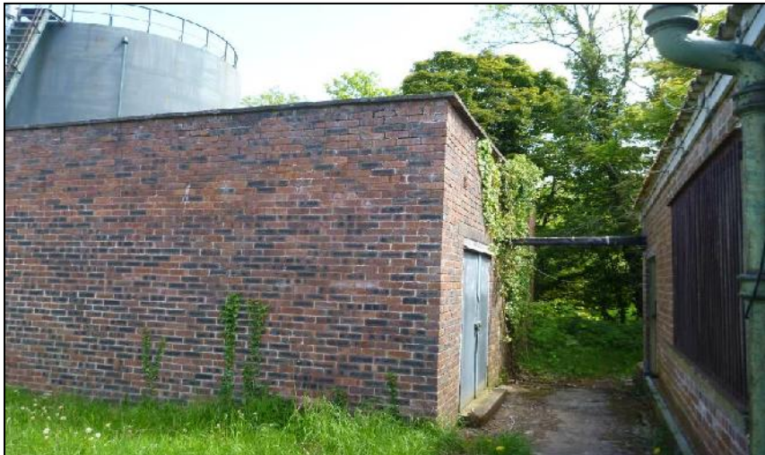
Photo 14: External boiler house for factory in east of the site, near to the river, with water tank beyond
