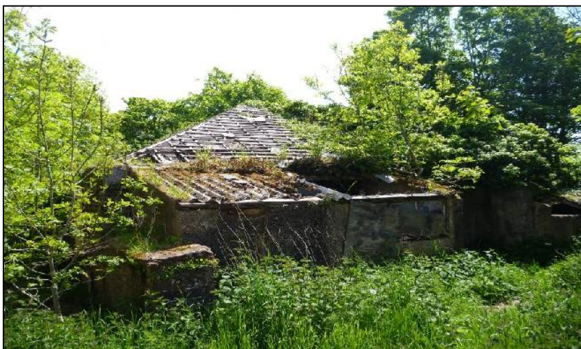
Photo 11: Derelict building in far south, heavily vegetated with trees beyond, down to the river
