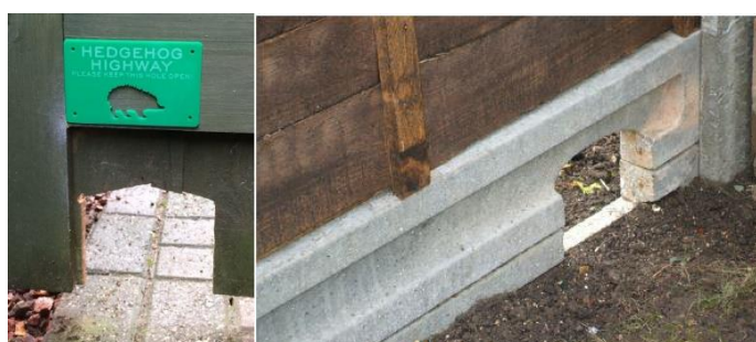
Insert 1: Showing wildlife access gap within fencing
