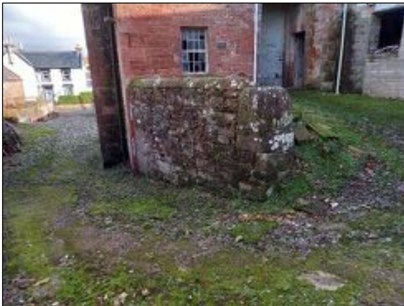
Plate 24: Detail of stone revetment wall which defines the north side of the ramp into the main entrance of the bank barn
