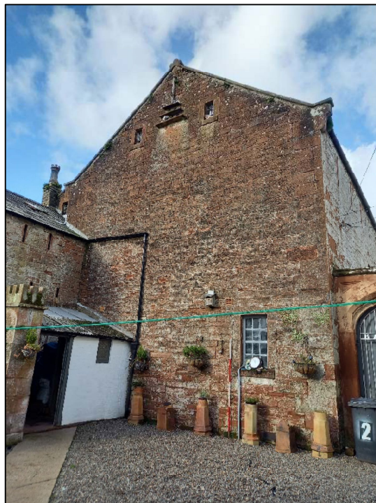
Plate 20: South elevation of the barn (Scale = 2m)
