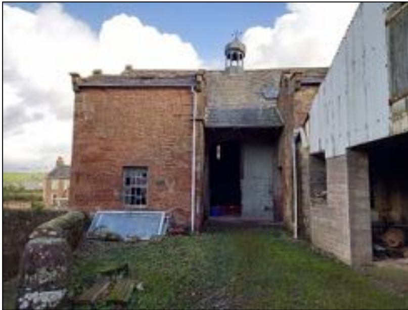
Plate 25: West elevation of the barn
