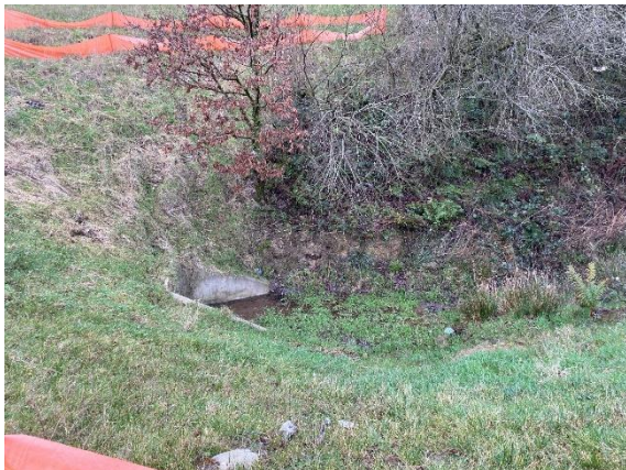
Photograph 5 – Outflow at southern end of ditch
