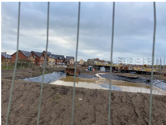
Photograph 20 – Construction site pond
