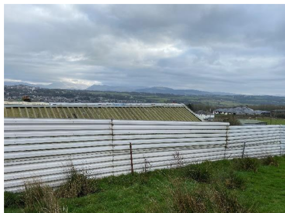
Photograph 11 – Western aspect of land grab fencing
