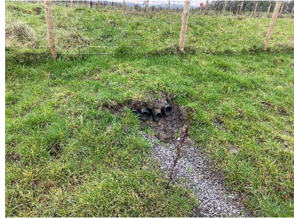
Photograph 19 – Overflow pipes from offsite pond
