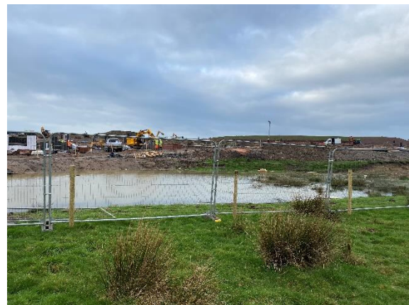
Photograph 21 – Construction site pond
